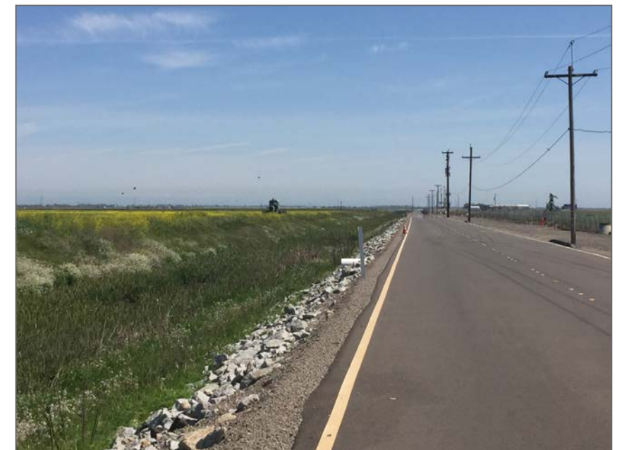
Looking east along Gibson Road from Road 102
