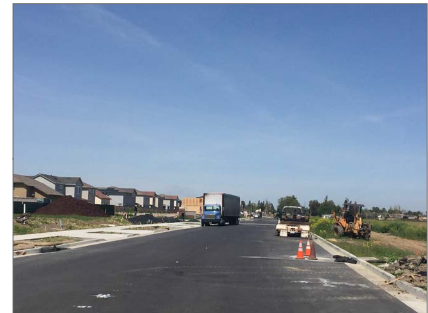
New housing development construction in northern portion of Harry Lorenzo Ave
