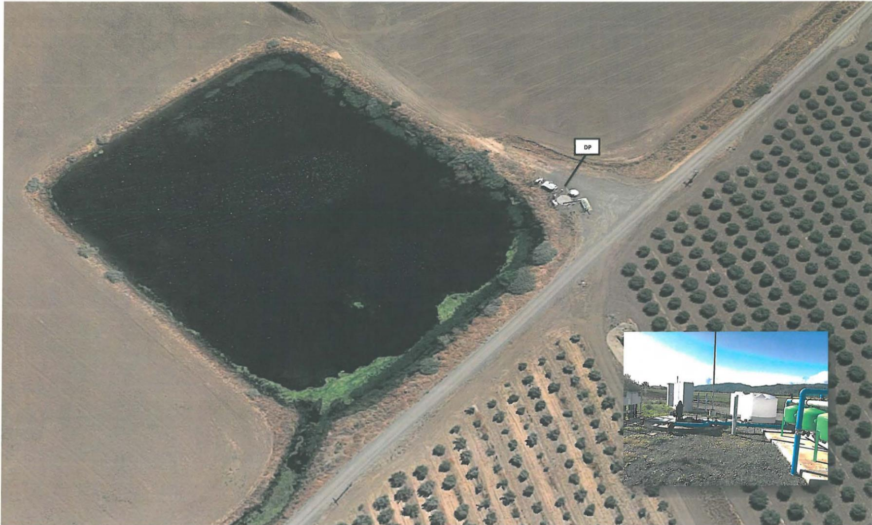
DP – Diversion Pump, State Highway 16, Brooks, CA 95606
