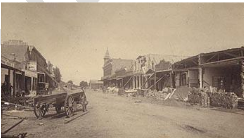
Figure 31: Downtown Winters after the 1892 Vacaville-Winters Earthquake
