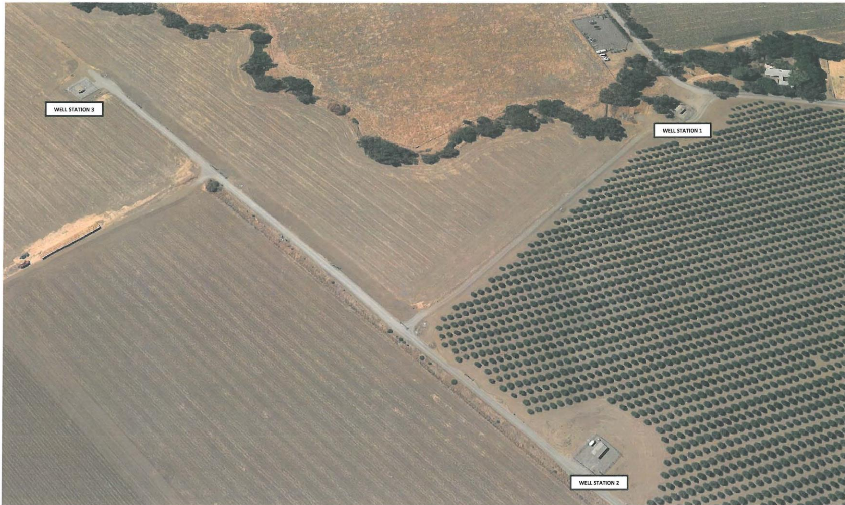
WS1 – Well Station 1 Pumphouse, 14300 State Highway 16, Brooks, CA 95606 - 266 SQ. FT. WS2 – Well Station 2 Pumphouse, 14100 State Highway 16, Brooks, CA 95606 - 350 SQ. FT. WS3 – Well Station 3 Pumphouse, 14600 State Highway 16, Brooks, CA 95606 - 250 SQ. FT.
