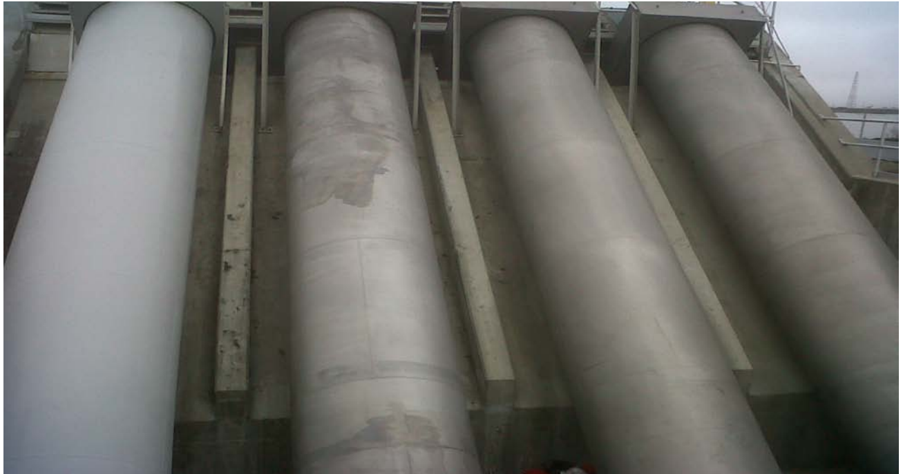
3 New Stainless steel Influent screw pumps installed at the head works.
