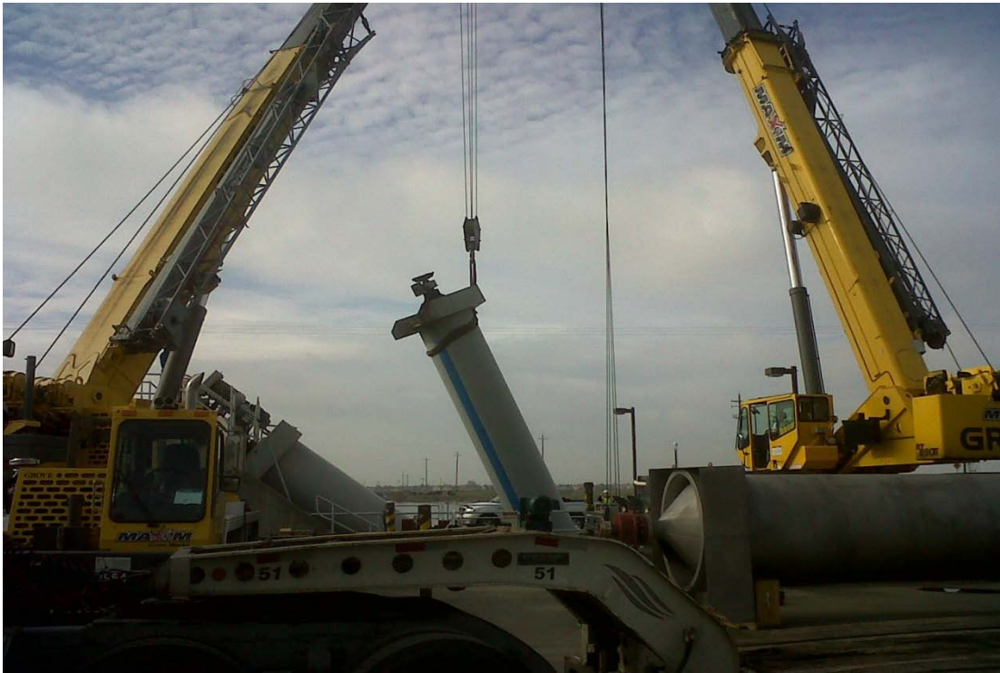
Draining the sewage out of Pump #3 before it is removed.
