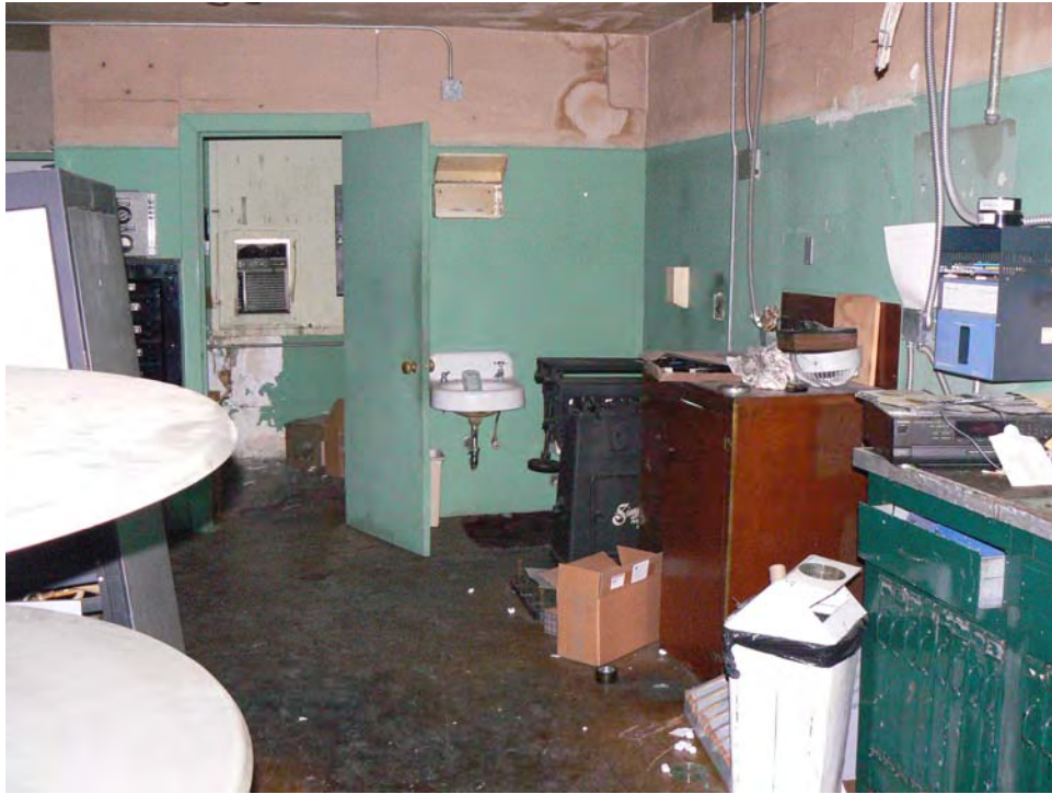
65. Projection Room - North and East
