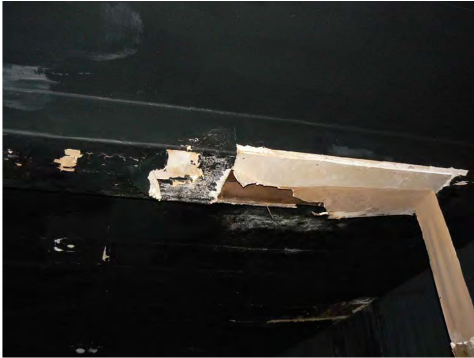
25. West Theatre - Beam and Ceiling Condition
