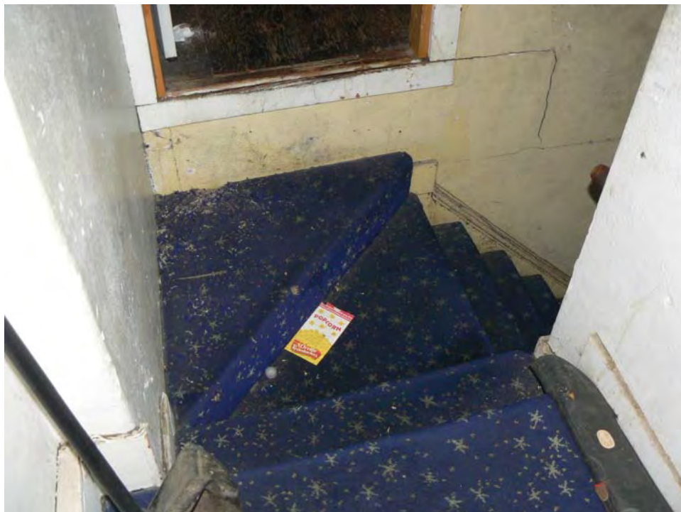
38. Stair to Mezzanine Storage and Offices
