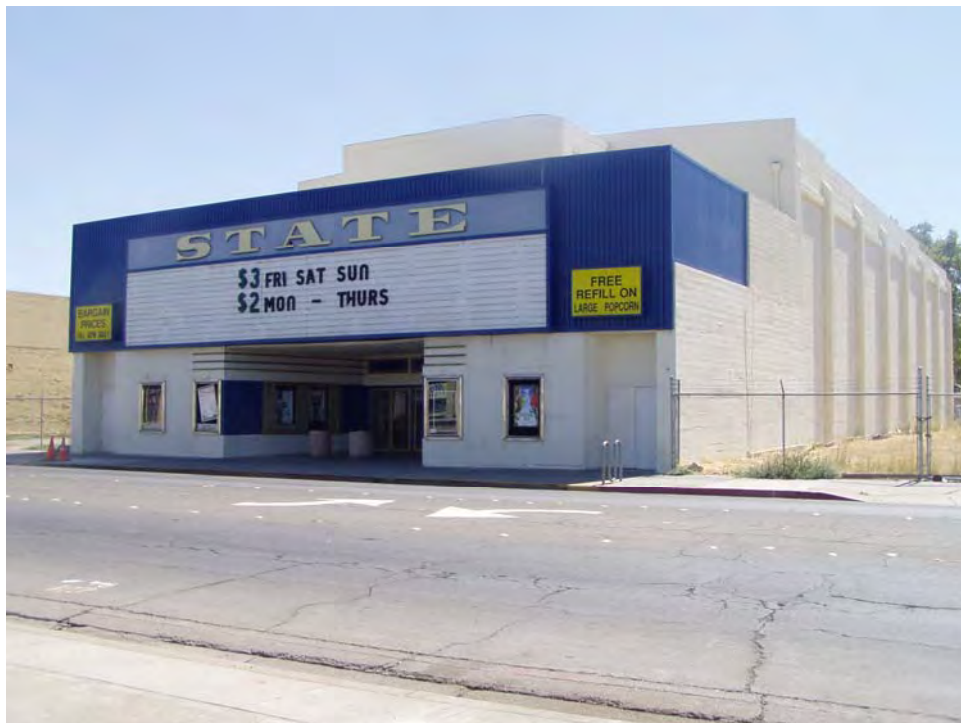
2. North Façade (Main Street)
