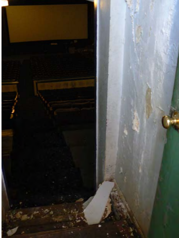
69. Projection Room - Wall Condition
