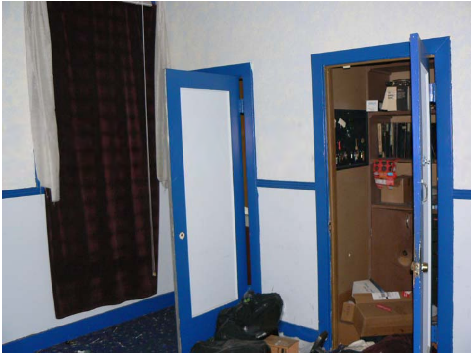
43. Mezzanine - Manager's Room
