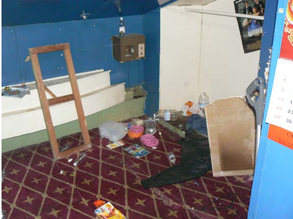
39. Mezzanine Center Storage Room
