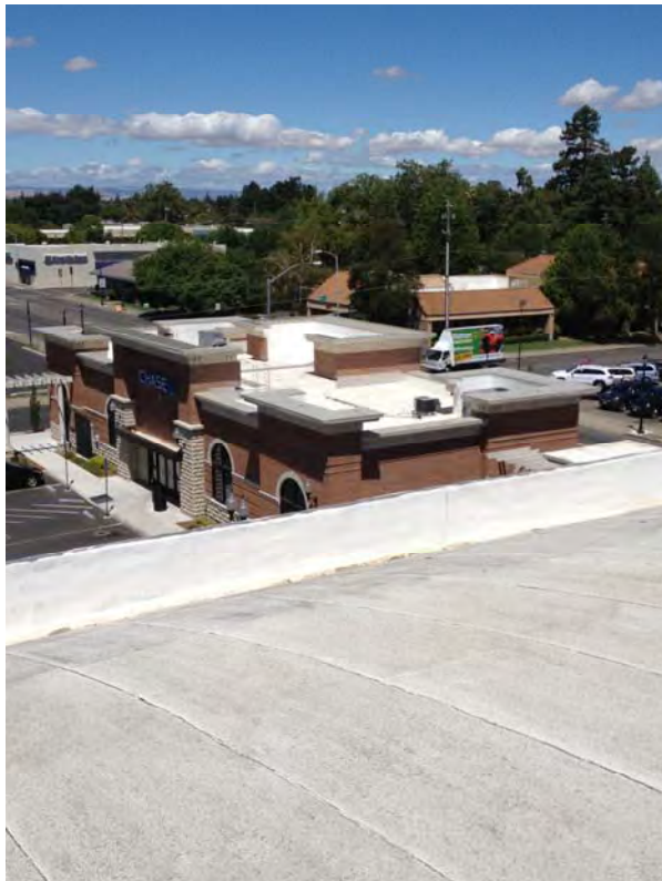
81. Roof - Main Roof Parapet
