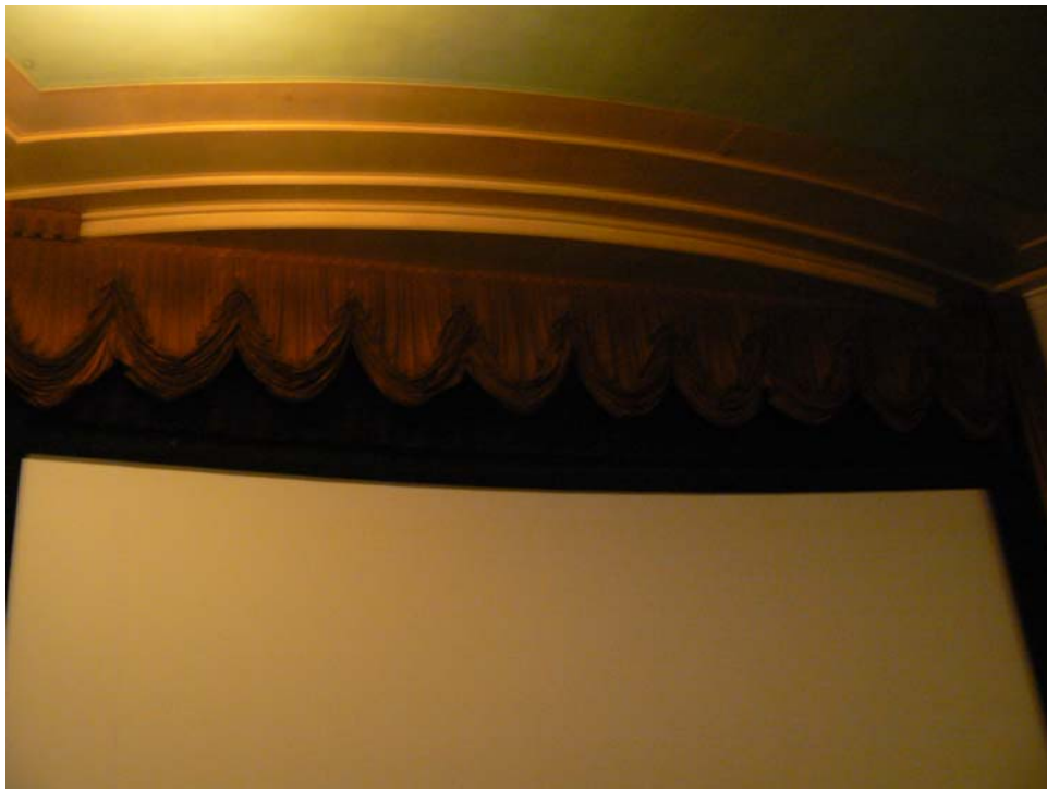
54. Auditorium Stage Curtain
