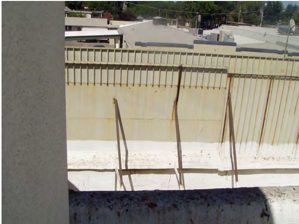
73. Roof - Back of Marquee
