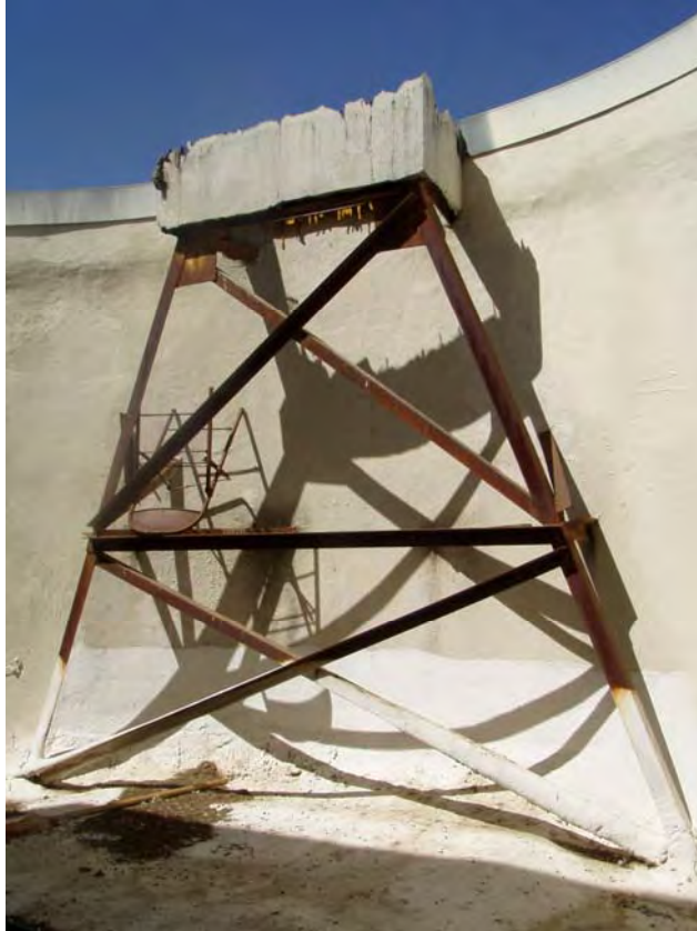
76. Roof - Back of Marquee
