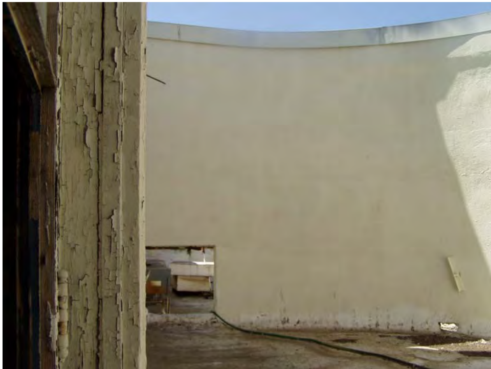
75. Roof - Parapet Opening
