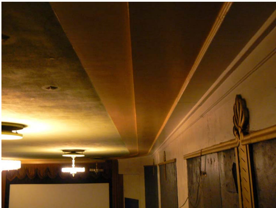
62. Auditorium - Ceiling Detail and Molding
