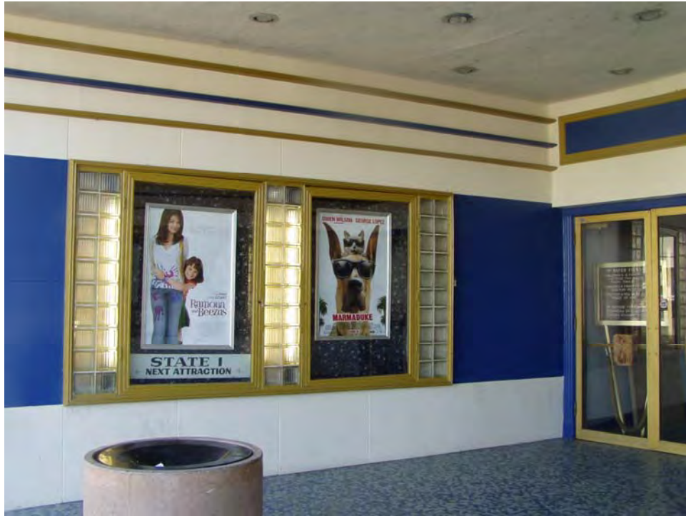
7. Entrance and Displays - East
