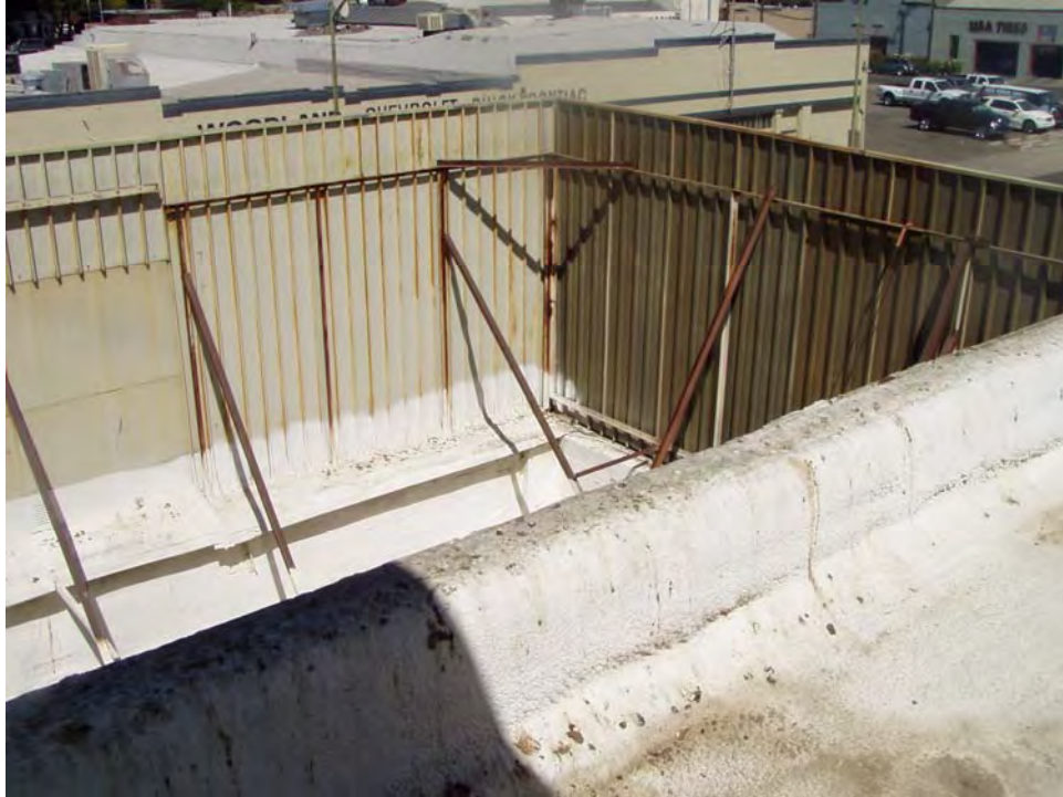
72. Roof - Northeast Corner
