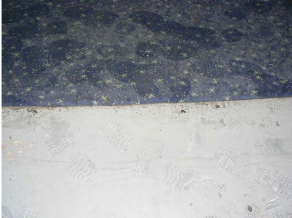
57. Auditorium - Floor Transition
