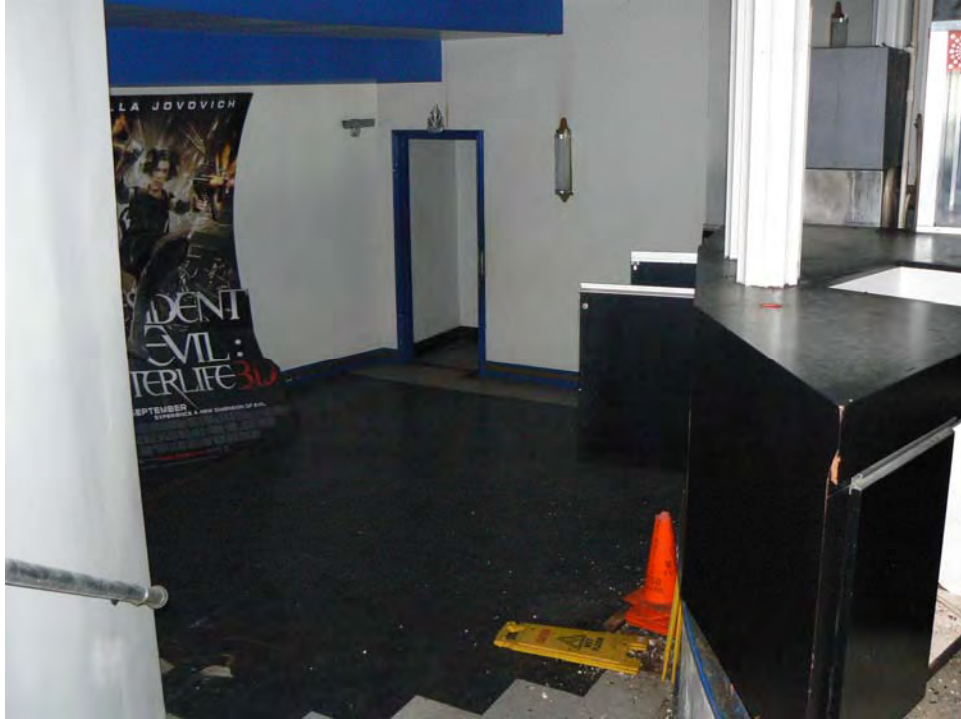
33. Hall to Rest Rooms
