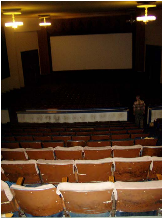
48. Auditorium Seating and Stage
