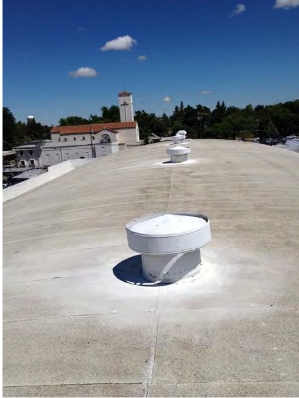
80. Roof - Main Auditorium Roof
