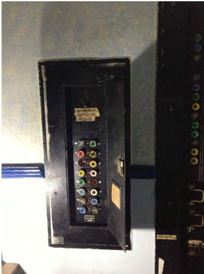
89. Existing Panel in Projection Room
