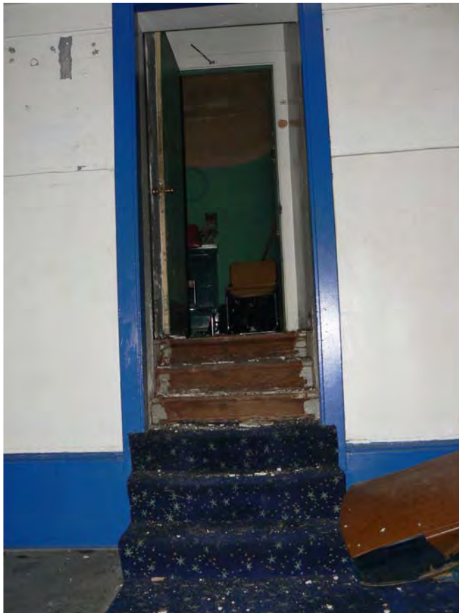
64. Auditorium - Projection Room Stair
