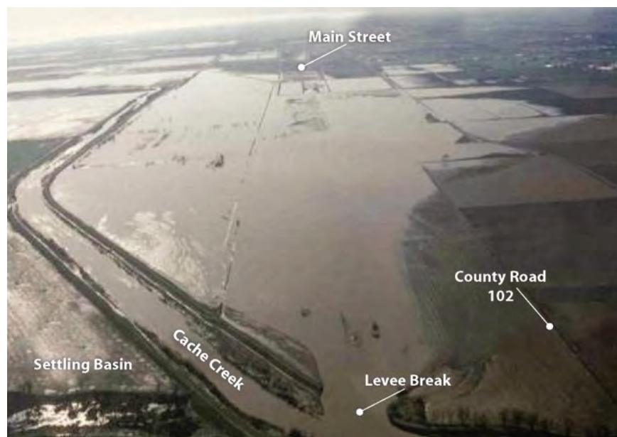
Due to inadequate flood infrastructure, major storms can result in significant flooding in the Woodland Planning Area—including in areas that have commercial, industrial, and residential development.
