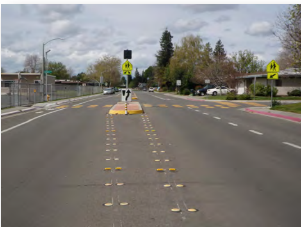
Enhanced Crossing with Beacon
