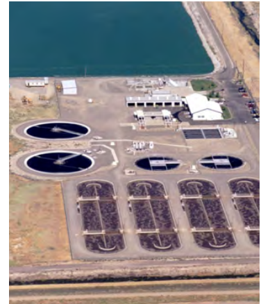
The Woodland Water Pollution Control Facility, located in the southeastern portion of the Planning Area, will have ample capacity for treating wastewater when upgrades to address solids treatment are complete (underway; anticipated completion in 2016).
