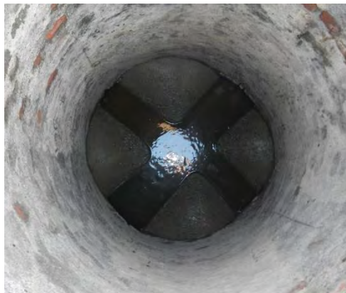
Manhole bottom after:
