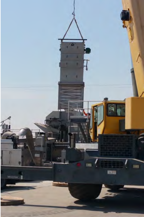
Bar Screen Installation
