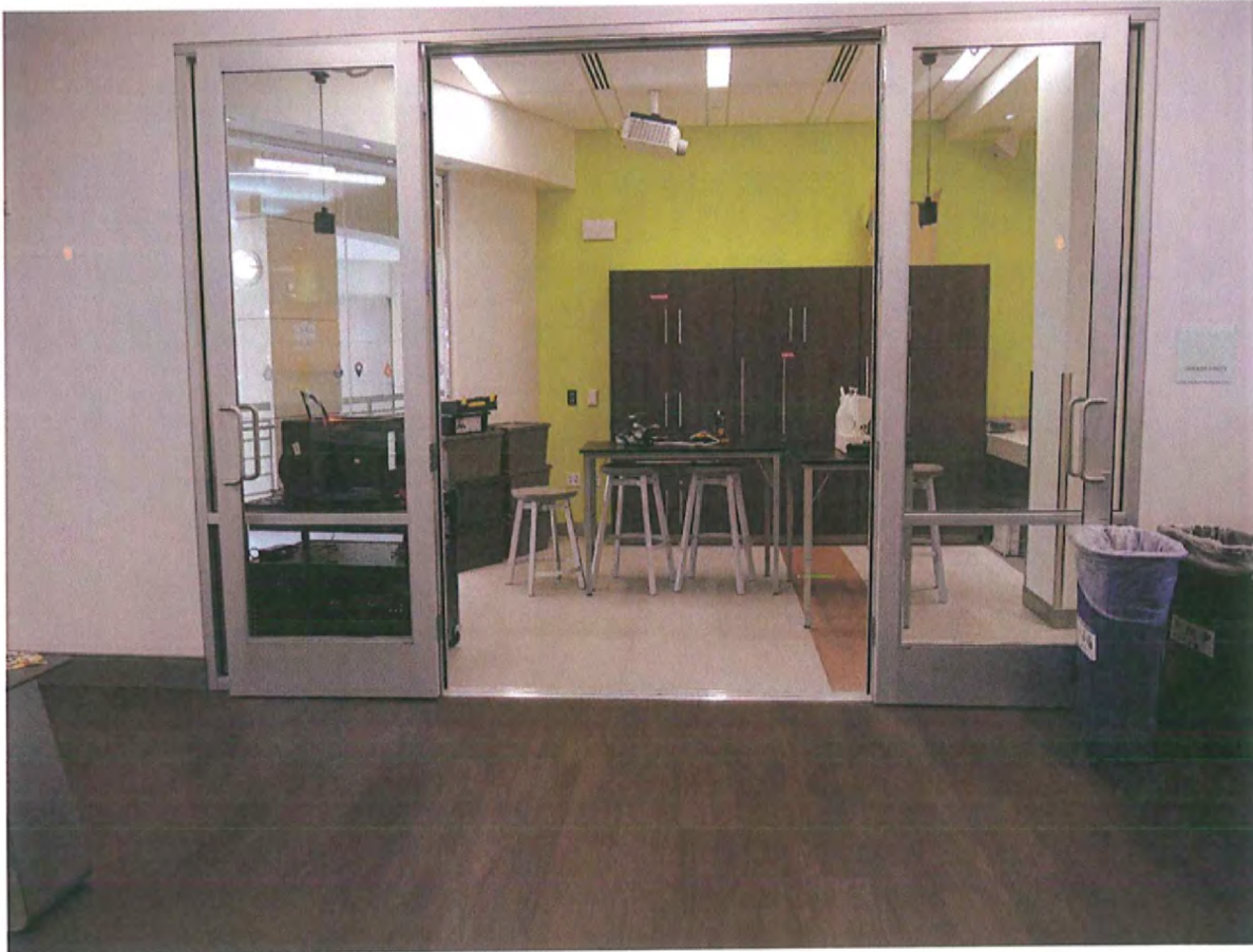
Figure 35 The Mix at SFPL Enclosed Make It Room
