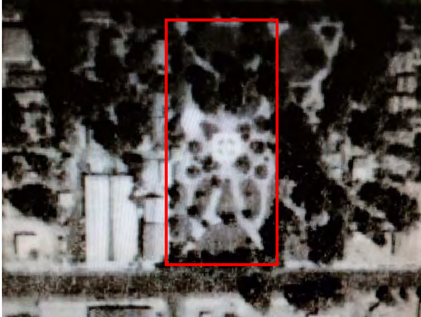
Figure 13: Aerial Photograph of Freeman Park, 1937, with the completed WPA landscape design (courtesy U.C. Davis Map Library).
