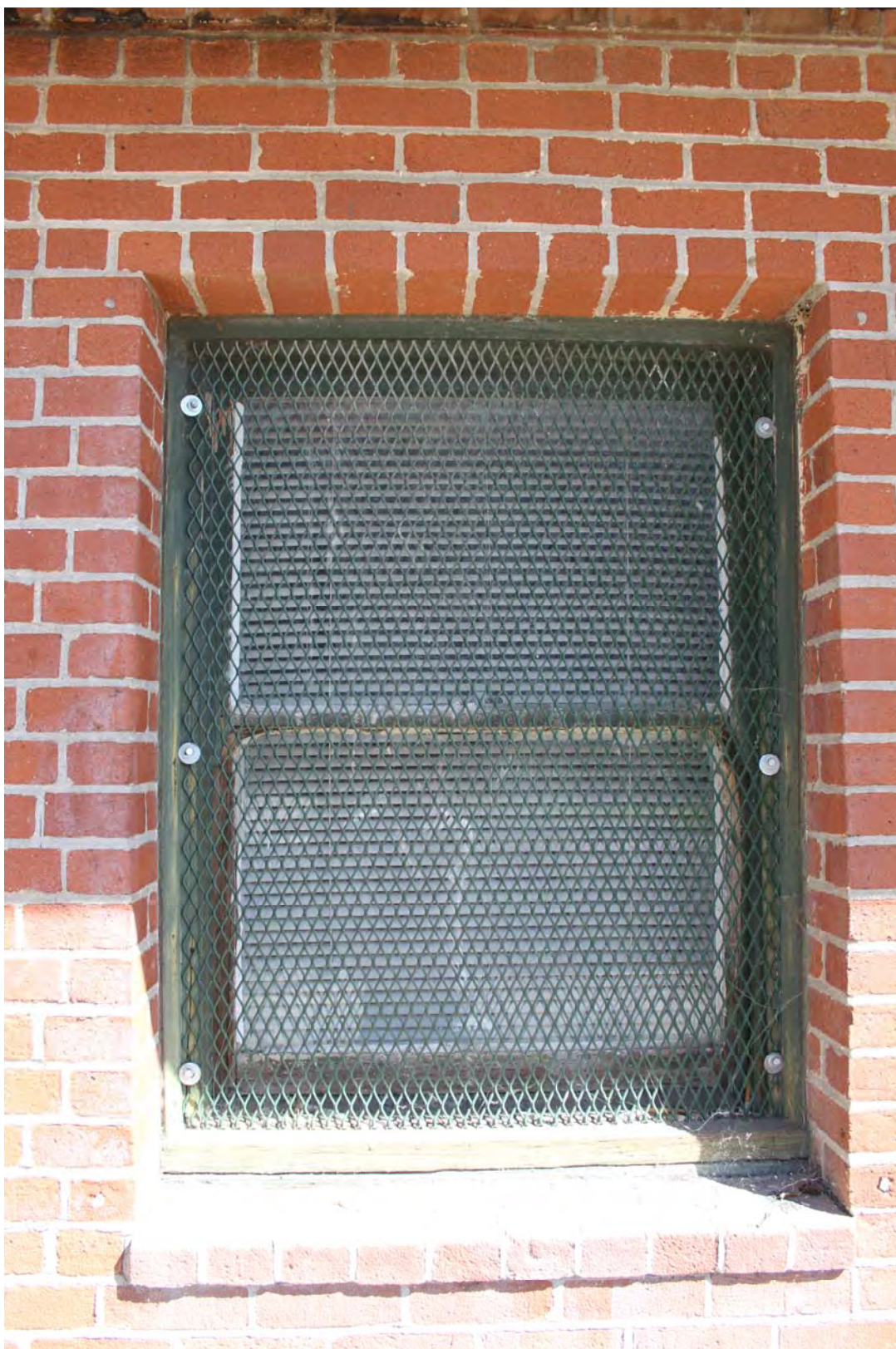
Photograph 11: Close-up of window details showing the double-hung windows covered by contemporary security screens.
