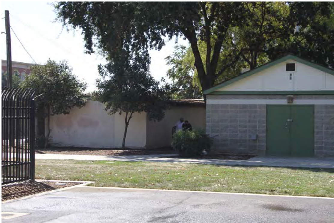
Photograph 19: View looking southwest from the rear parking area towards the Freeman Park restrooms and the rear of 1017 Main Street.
