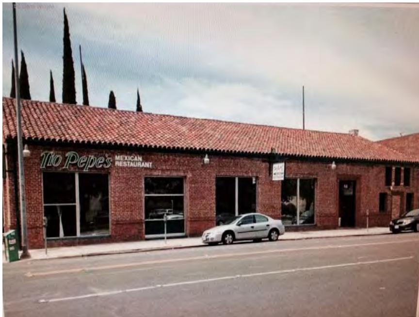
Figure 6: Former DMV office, 411 N. Hunter Street, Stockton, CA.
