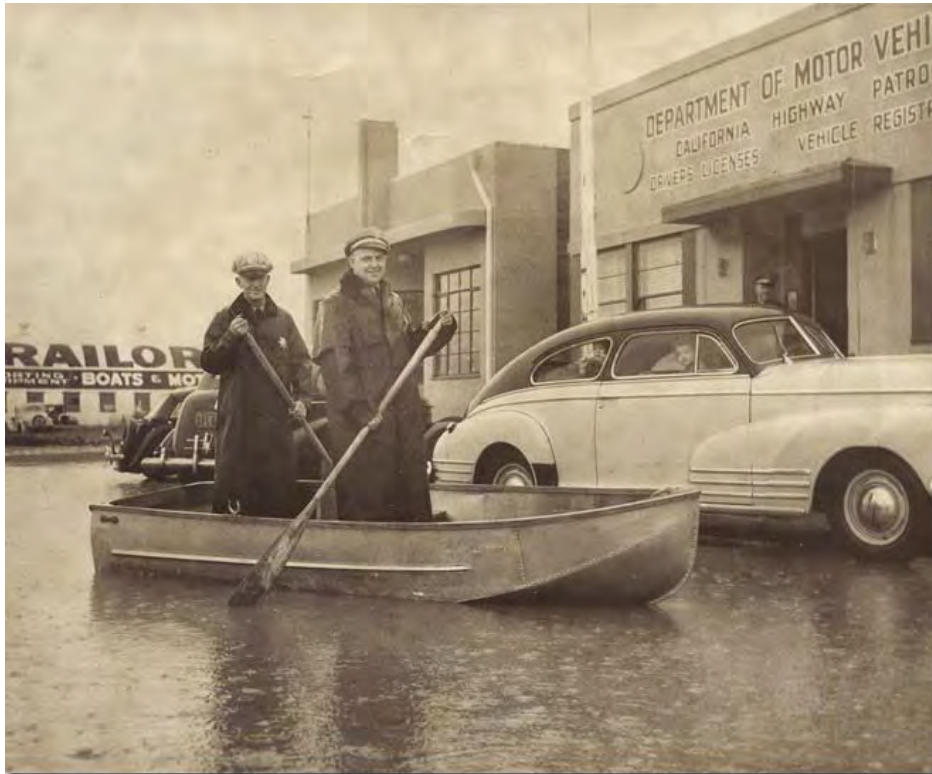
Figure 7: Former shared DMV and Highway Patrol Office, San Rafael, CA, during the flood of 1945.
