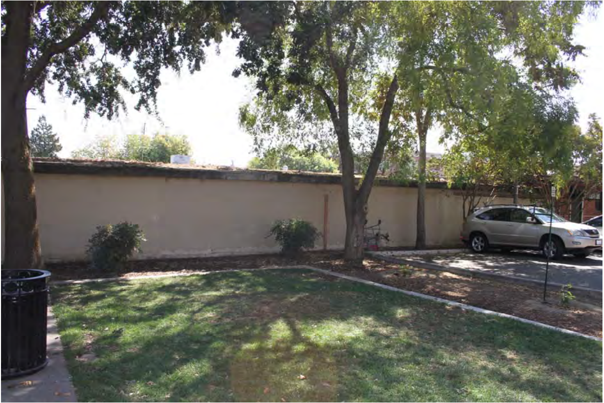
Photograph 20: View looking east at the west elevation of the addition to 1017 Main Street.
