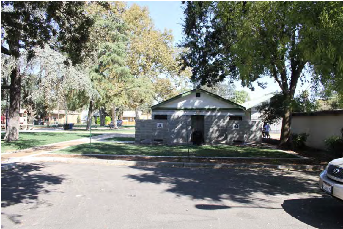
Photograph 6: View looking north at Freeman Park restrooms and 1017 Main Street on the right.
