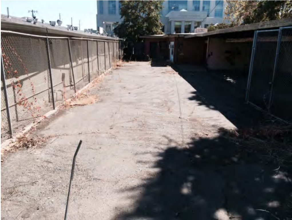
Photograph 22: View looking south inside the gated and fenced courtyard behind 1017 Main Street. The carports or bays on the right are later additions.
