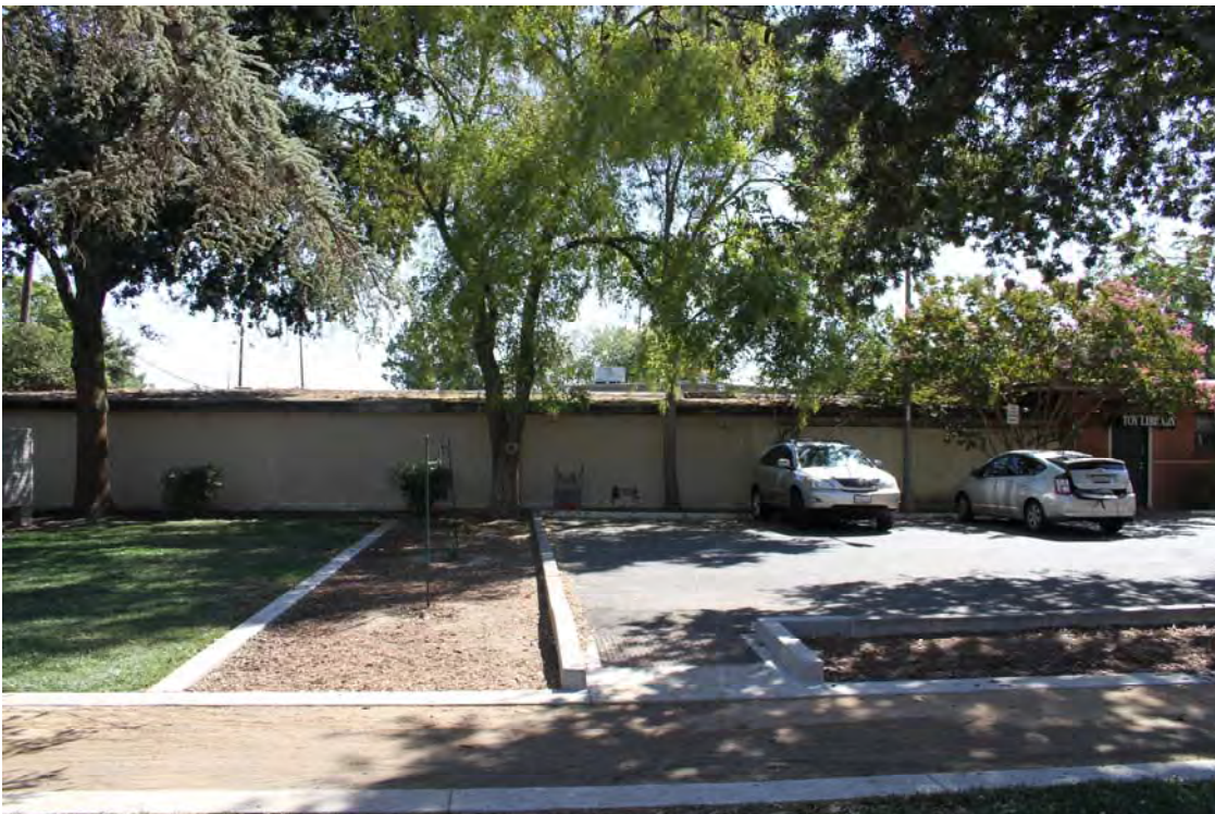
Photograph 15: View looking east from Freeman Park at the rear addition (parking bays) for 1017 Main Street. The addition was completed after 1949-1950.
