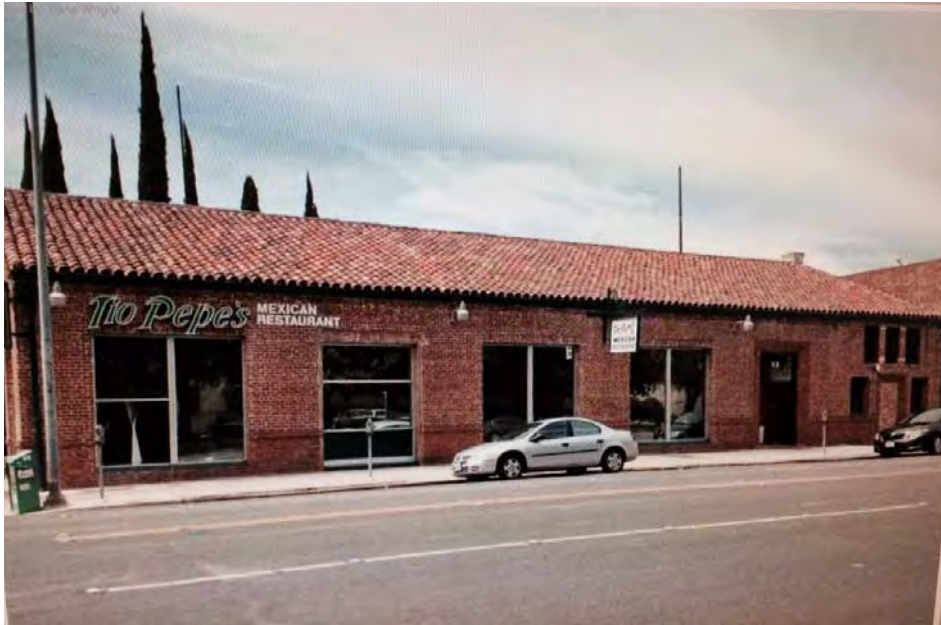
Figure 22: Former DMV office, 411 N. Hunter Street, Stockton, CA.
