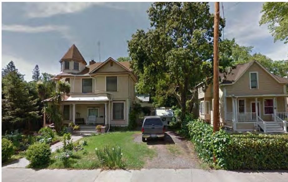
520 Second Street, looking west. One of the key characteristics of the Queen Anne residence is its asymmetric design. Note the offset porch to the left and the tower as compared to the older Late Victorian symmetrical design to the right.
