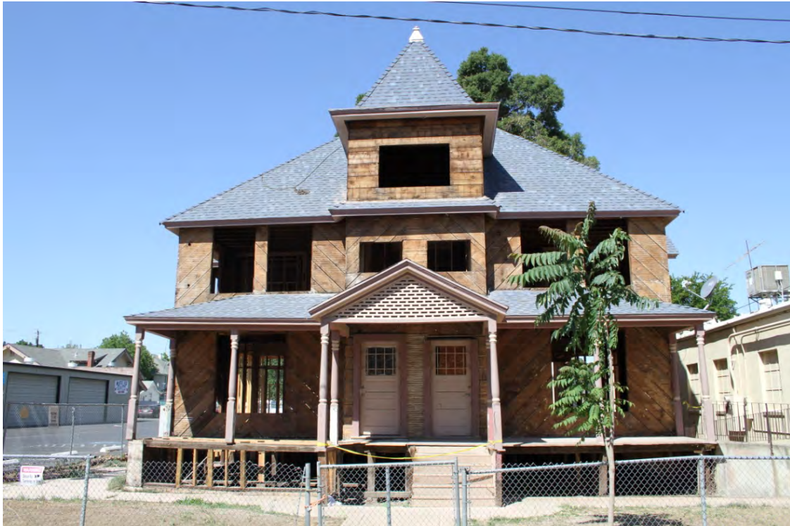
FIGURE 4: View looking west at 440-442 College Street
