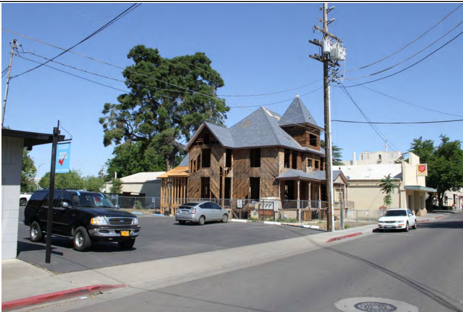
15. View looking northwest at the subject property from College Street.
