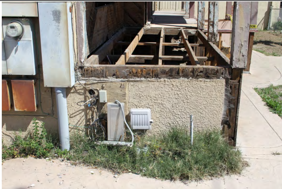
9. View looking at the footing below the front porch and the old stucco wall cladding.
