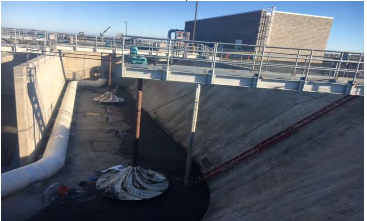
Basin 4 cleaned out for contractor to finish punch-list items
