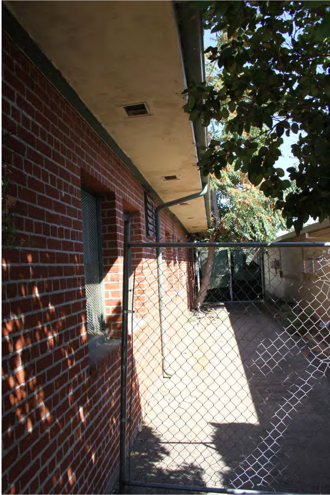
Photograph 9: View looking north at the east elevation of 1017 Main Street. The building on the right is the Budget Inn, located at 1021 Main Street.
