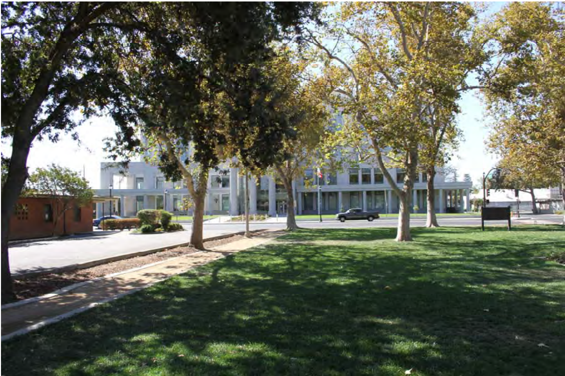
Photograph 17: View looking south across the right or east side of Freeman Park towards the new County Courthouse.
