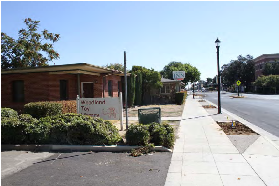
Photograph 5: View looking east down Main Street with 1017 Main Street on the left.
