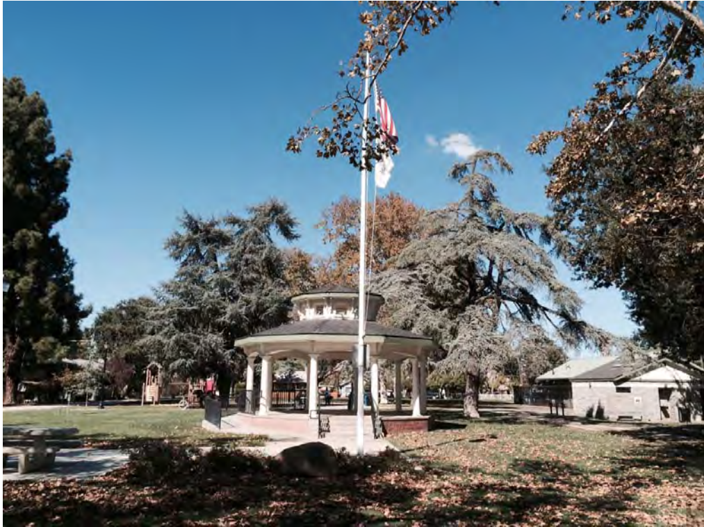
Photograph 26: Close-up of the gazebo in Freeman Park, built in 2001.
