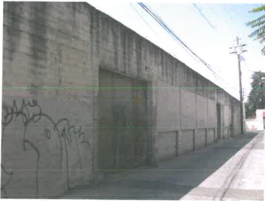
VIEW WEST - ALLEY FACADE
