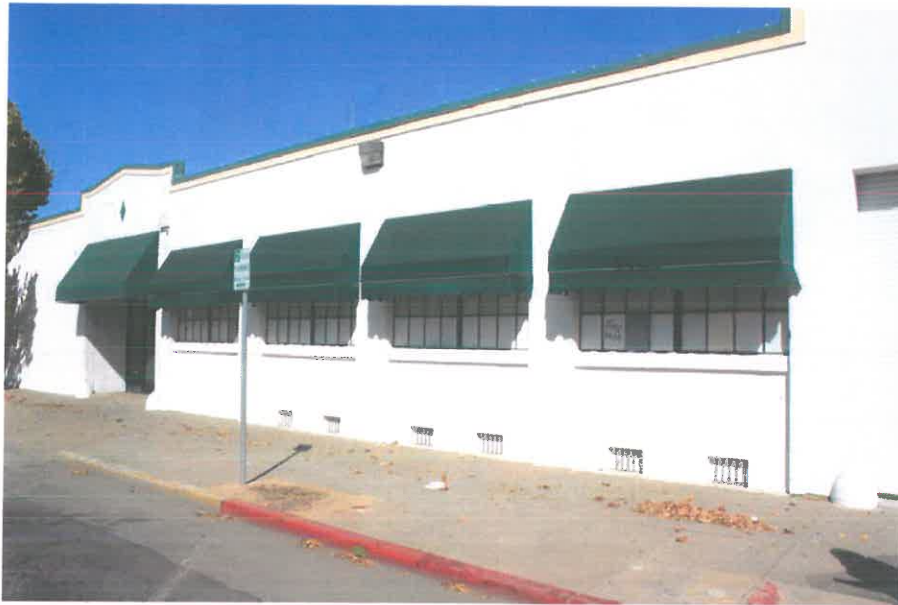
Figure 1 Partial South elevation, view northwest
