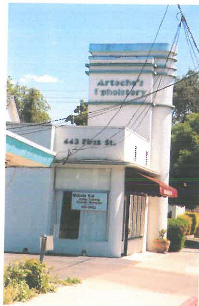
Mulcahey Building 443 1 st Street
