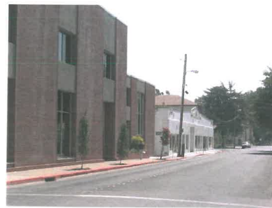
WDC BUILDING - NORTH OF PROJECT SITE
