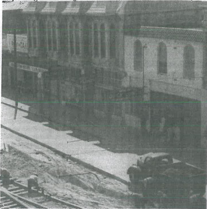
Clark and Beamer Place buildings on left with workers repairing Northern Electric train tracks
