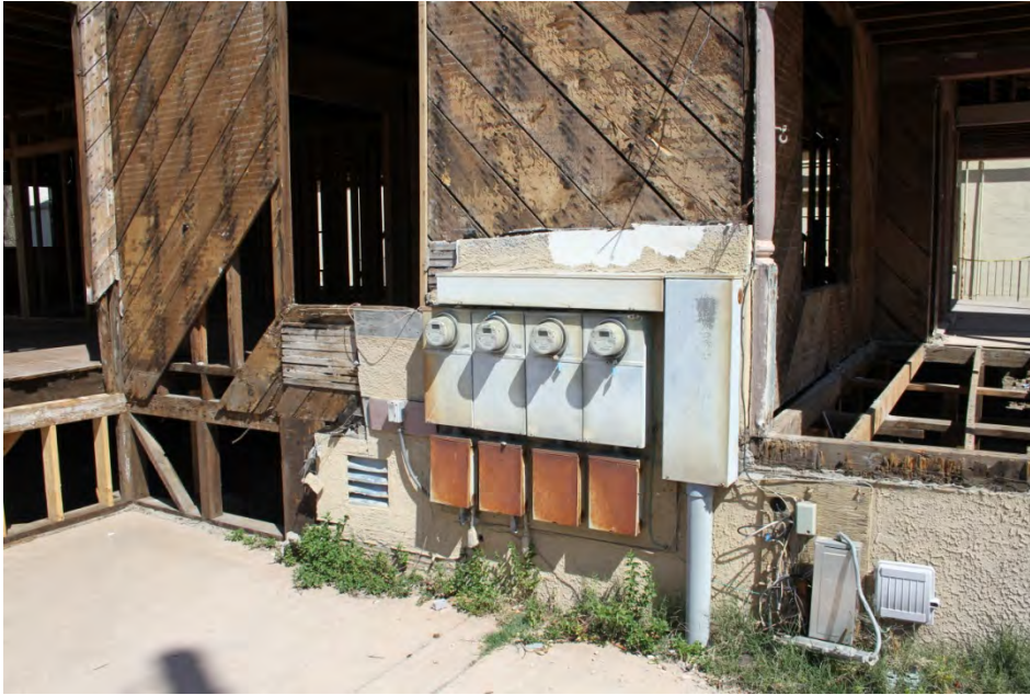
10. View looking north at the south elevation electrical boxes and sub-floor.
