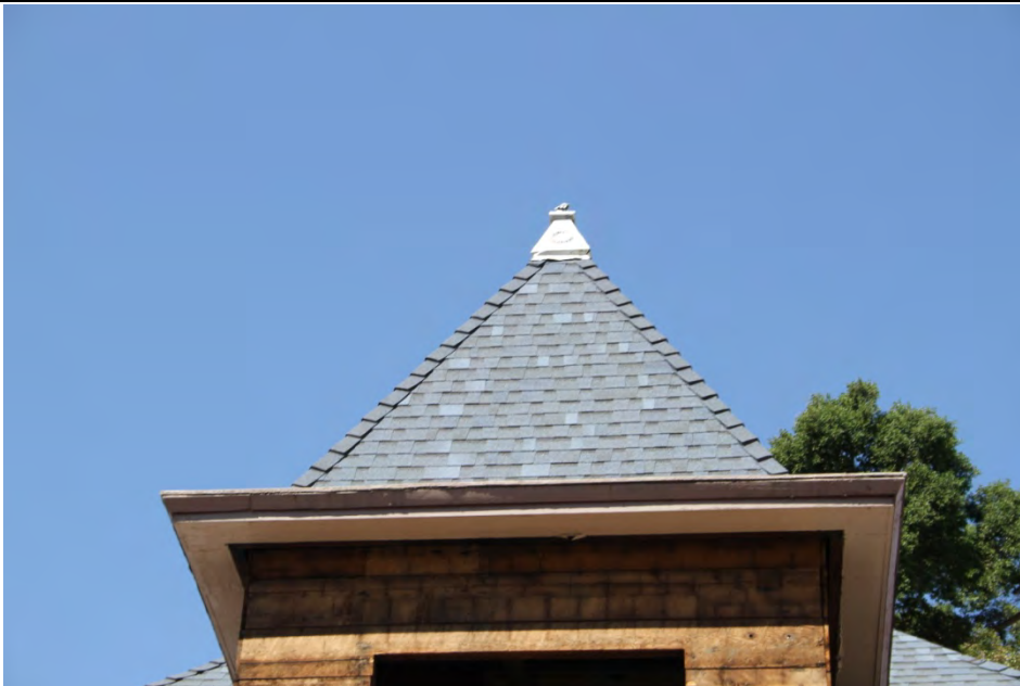
11. View looking at the top of the tower where the shingle siding existed until recently.
