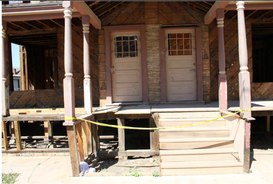
8. View looking west at the two front entry doors.
