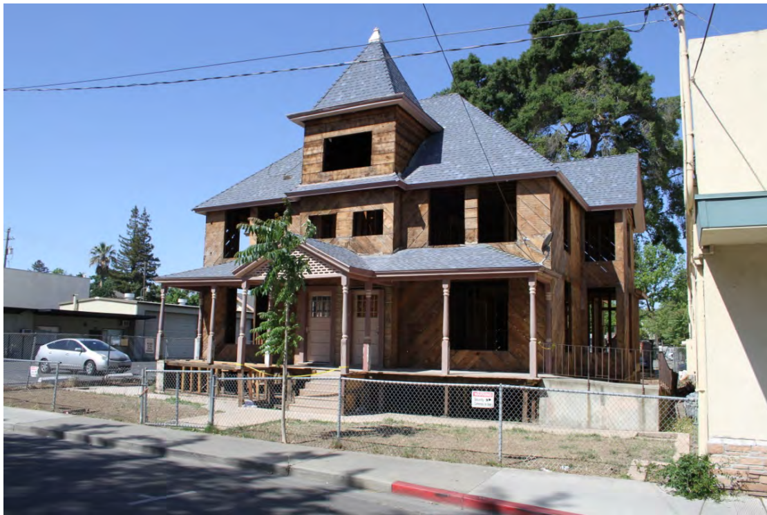
FIGURE 5: View looking southwest at 440-442 College Street
