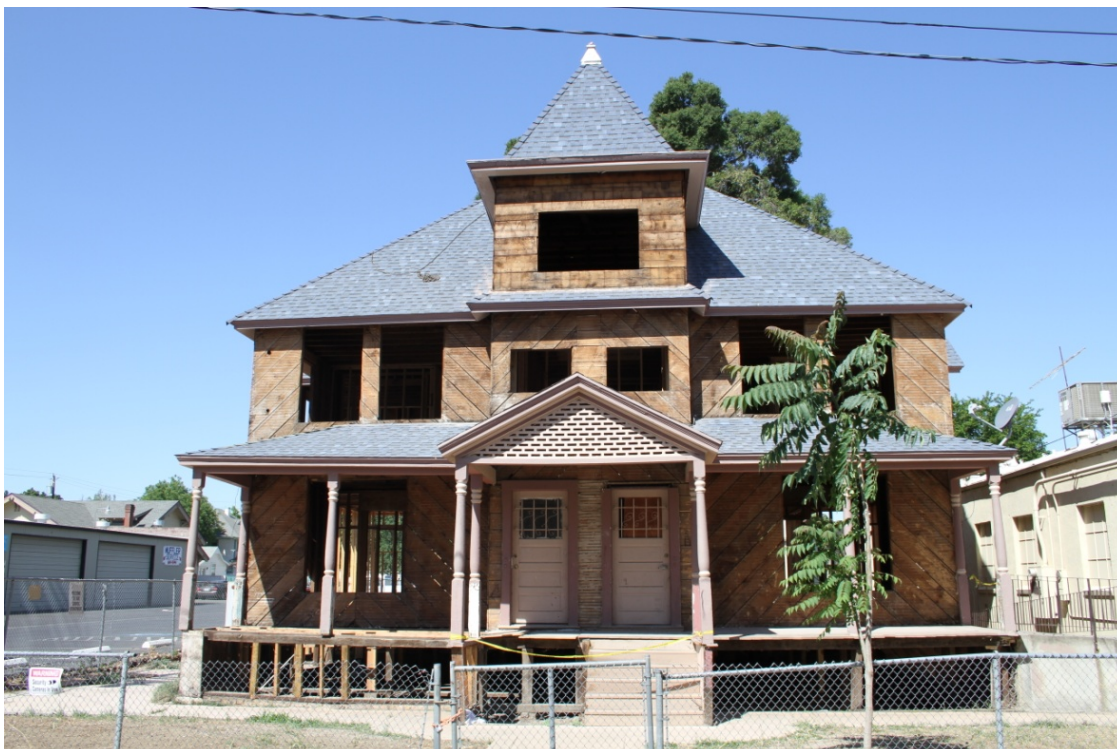
FIGURE 4: View looking west at 440-442 College Street
