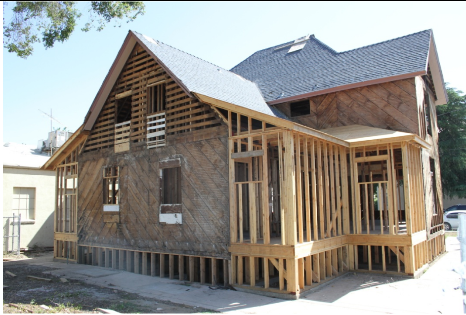
6. Closer view looking east at the west elevation.
