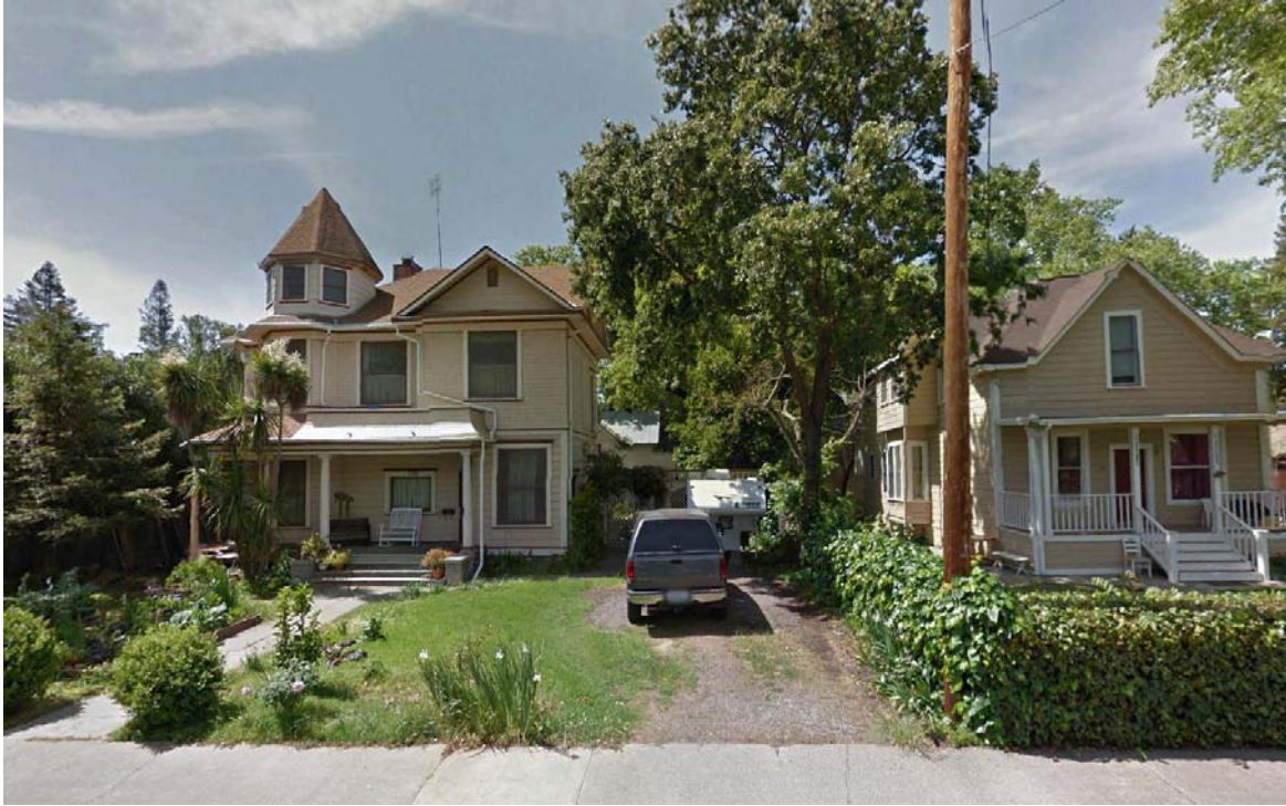
FIGURE 9: 520 Second Street, looking west. One of the key characteristics of the Queen Anne residence is its asymmetric design. Note the offset porch to the left and the tower as compared to the older Late Victorian symmetrical design to the right.
