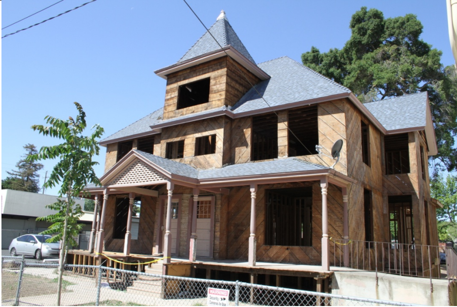
1. View looking west at 440-442 College Street from College Street.
