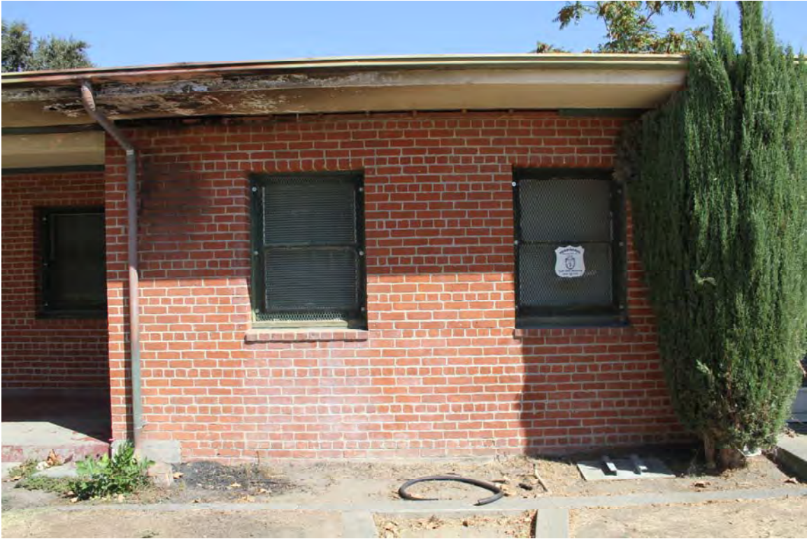
Photograph 7: View of the right front facade of 1017 Main Street showing brick and window detail.
