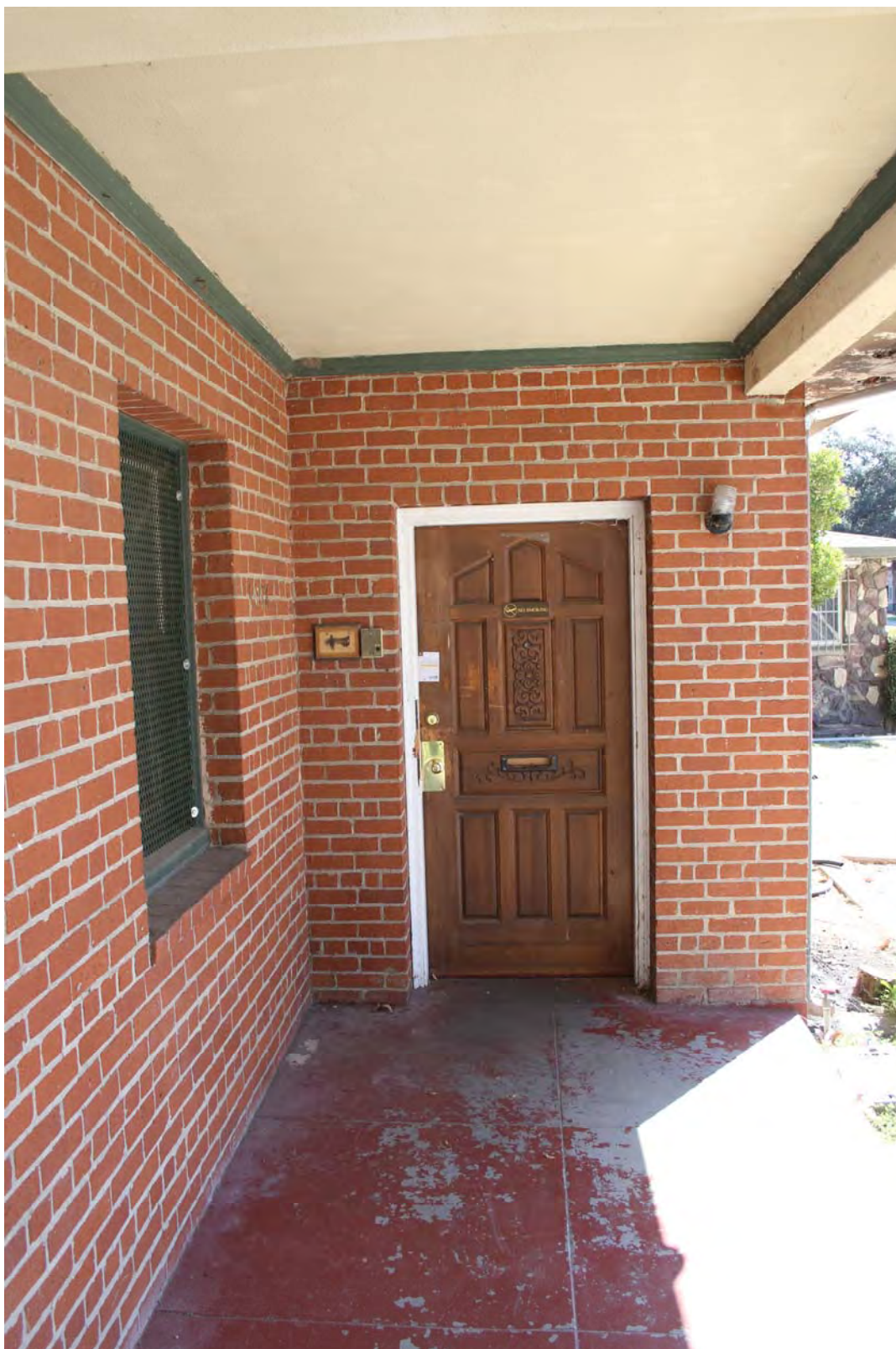
Photograph 10: View of the replaced front entry door, looking east.
