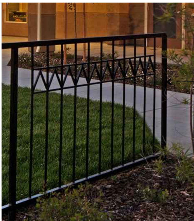
4'-0" TALL OPEN STEEL FENCE (GATE SIMILAR)
