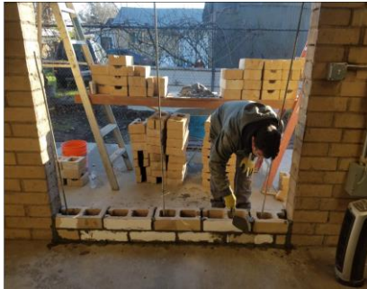
Everman brick laying
