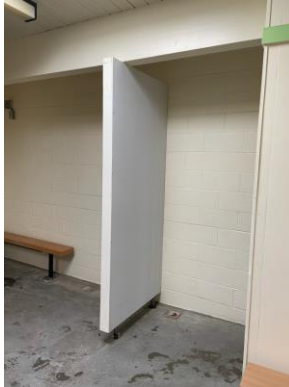
Privacy wall inside men's locker room
