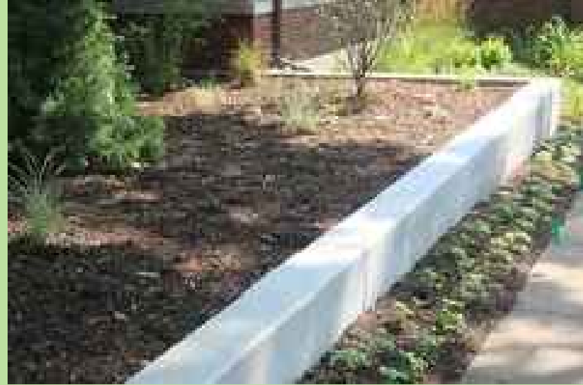
CONCRETE RETAINING CURB
