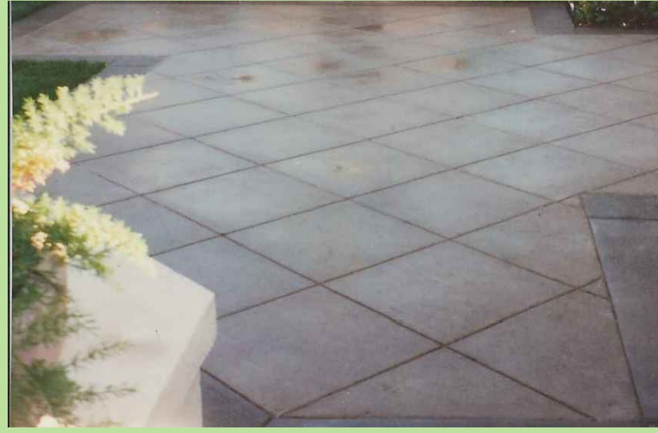
DIAGONAL SCORED CONCRETE PAVING
