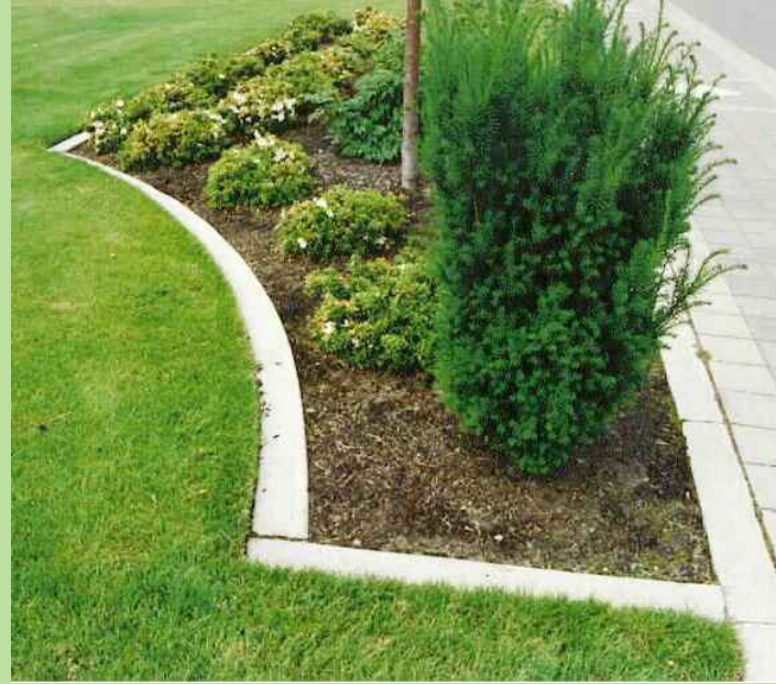
CONCRETE MOW CURB
