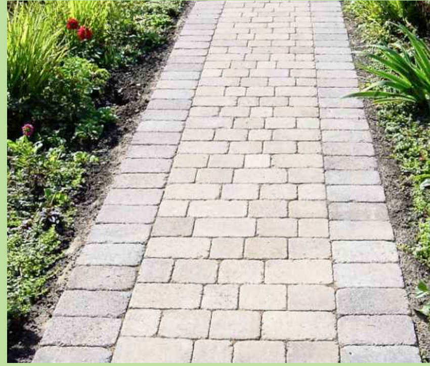
CONCRETE PAVER WALK
