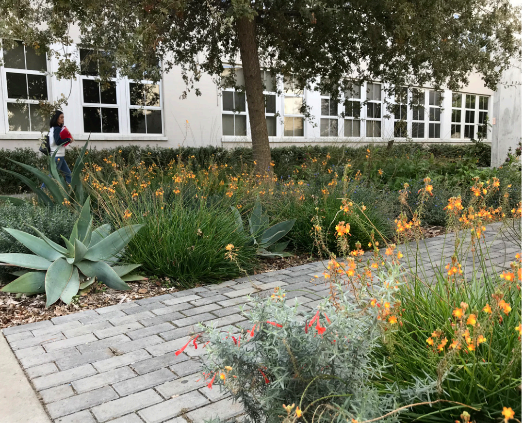
Pervious pavement pathway/patio space
