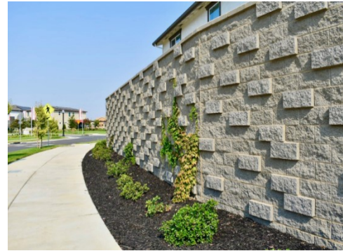
Vines and landscaping help soften retaining walls and masonry walls required for sound attenuation.
