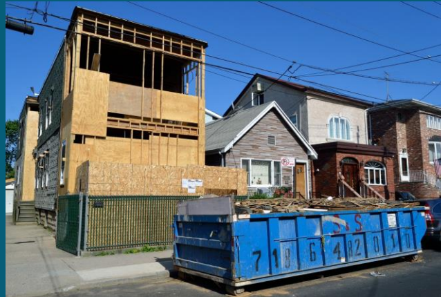
Construction & Demolition Ordinance
