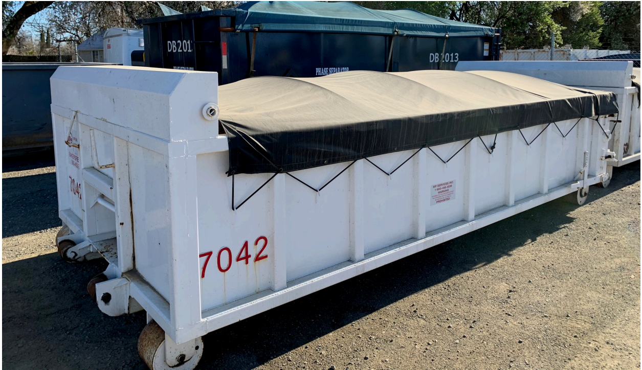
Covered roll-off bins for construction materials, debris and non-hazardous soils (close-up)
