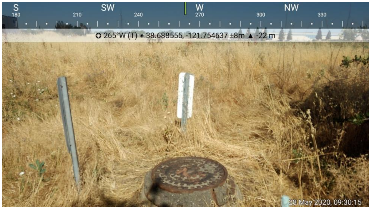
Photo 8: The storm drain manhole present in the southeastern corner of the Project site, looking west.
