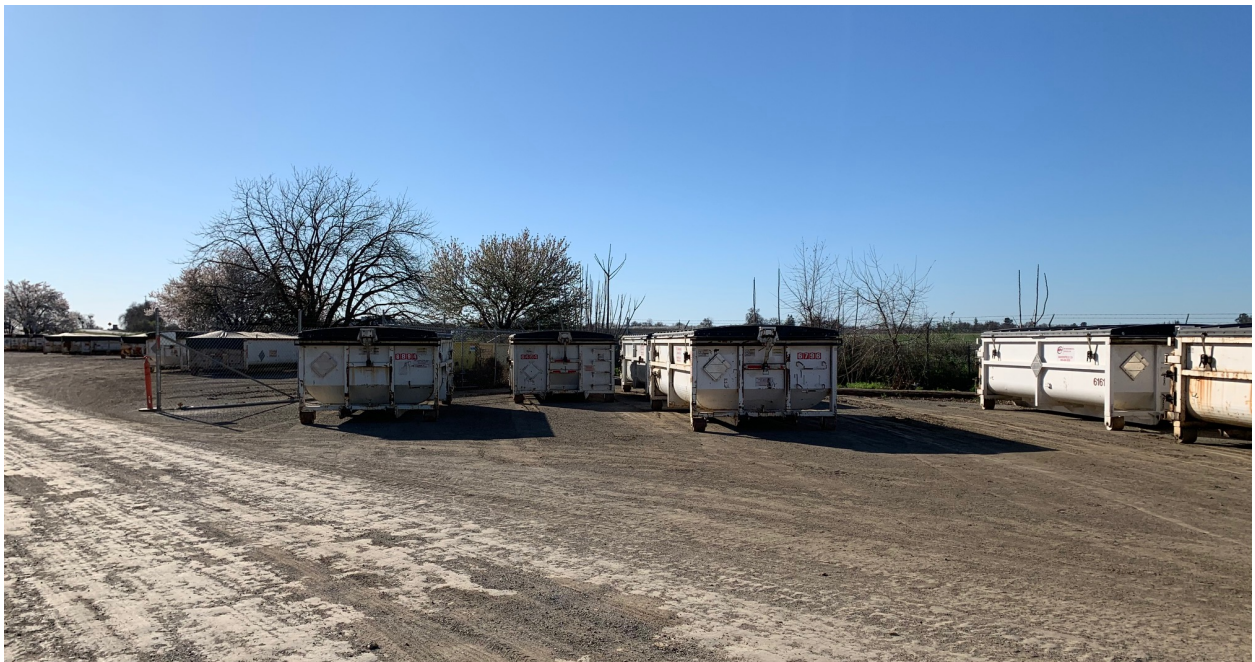
Covered roll-off bins for construction materials, debris and non-hazardous soils
