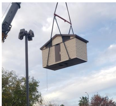
Manufactured restroom being lifted from the truck by a crane onto the concrete pad near Harris ballfield
