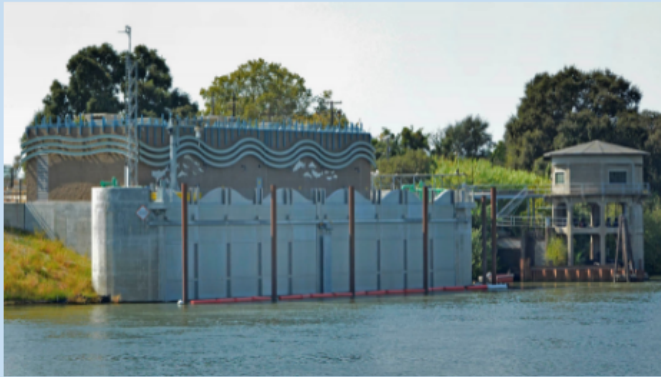
Sacramento River joint water new and old water intake facilities
