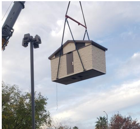
Manufactured restroom being lifted from the truck by a crane onto the concrete pad near Harris Park ballfield
