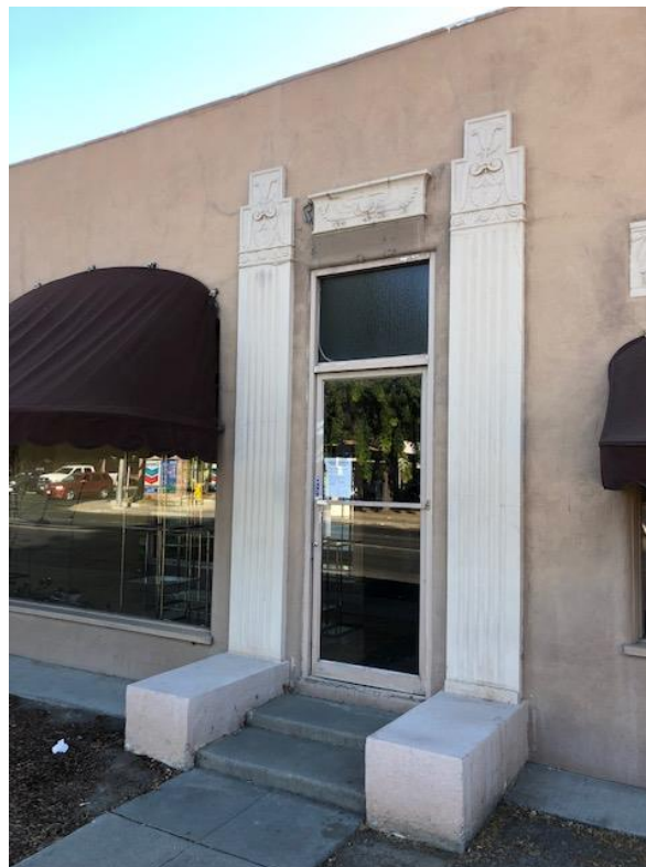
Photograph 10: View of the pilasters, Egyptian Revival stylized capitals, and frieze above the side door facing West Street.
