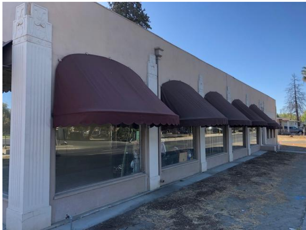
Figure 4: View looking south at the west elevation of 2 Main Street.
