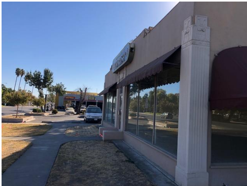
Photograph 4: View looking east at the front elevation of 2 Main Street.
