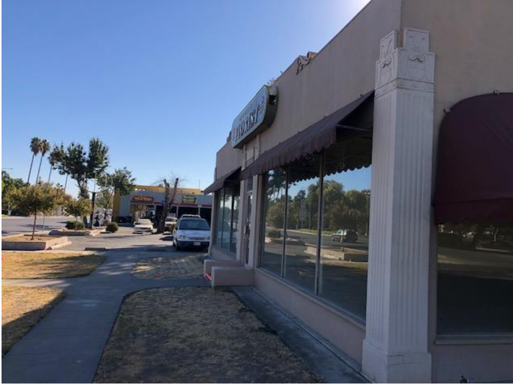
Figure 5: View looking east at the front or north elevation of 2 Main Street.
