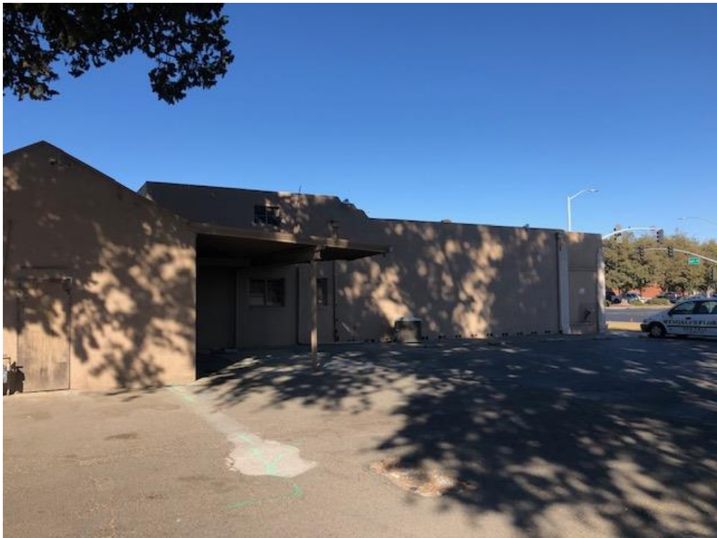
Figure 6: View looking west at the east elevation of 2 Main Street.
