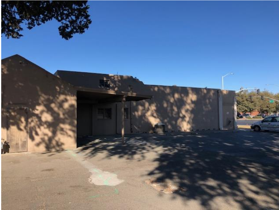
Photograph 7: View looking northwest at the east elevation of 2 Main Street. The two additions are on the far left. The original building is on the right.
