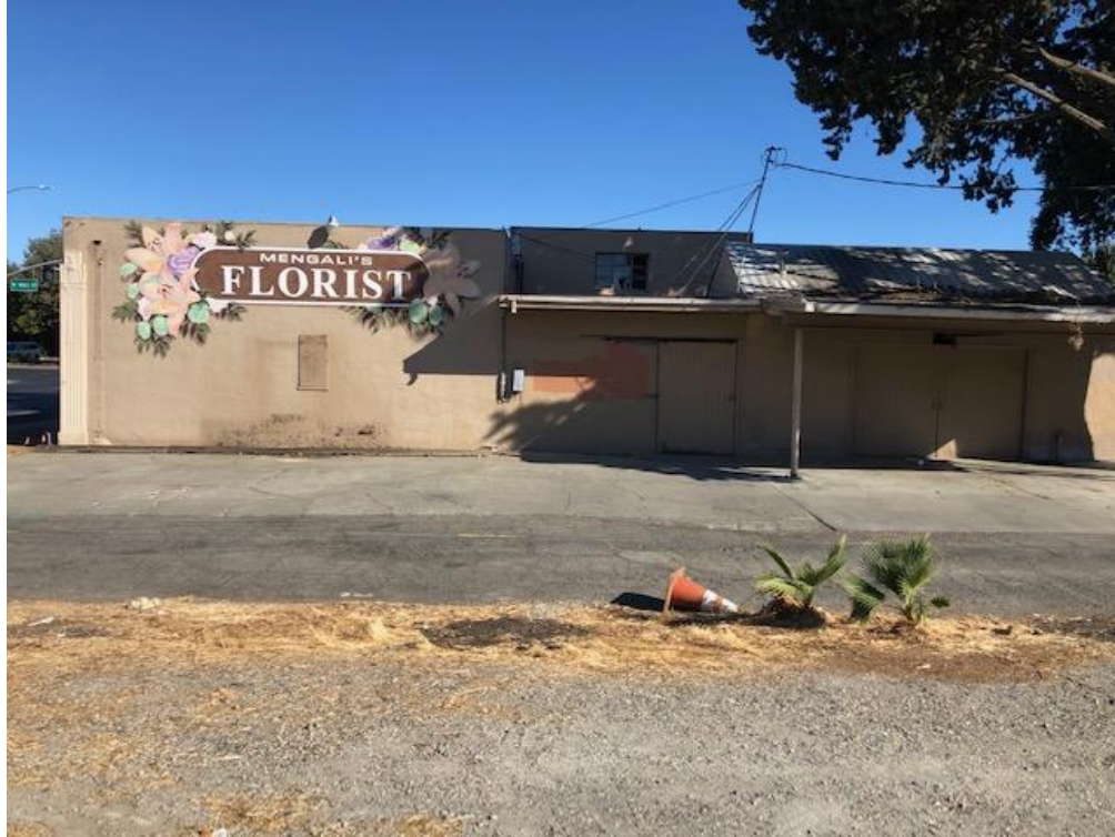
Figure 7: View looking north at the rear or south elevation of 2 Main Street.
