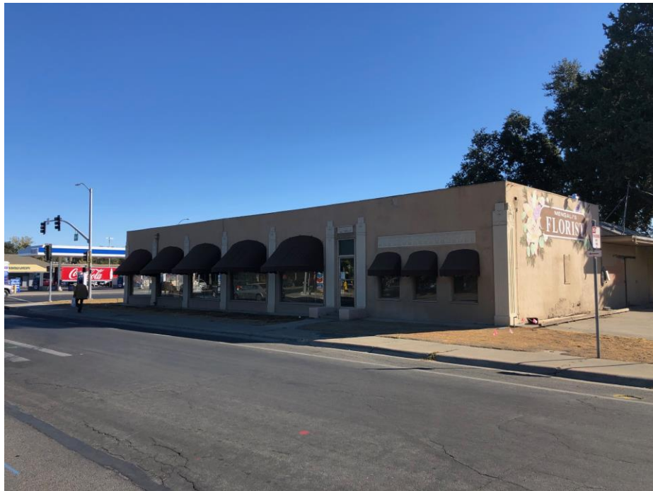
Photograph 2: View looking northeast across West Street at 2 Main Street.
