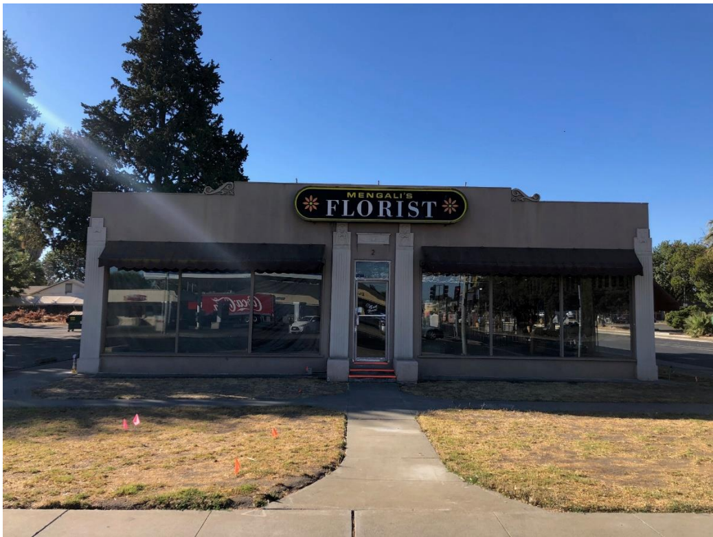
Figure 2: Front or north elevation of 2 Main Street looking south.
