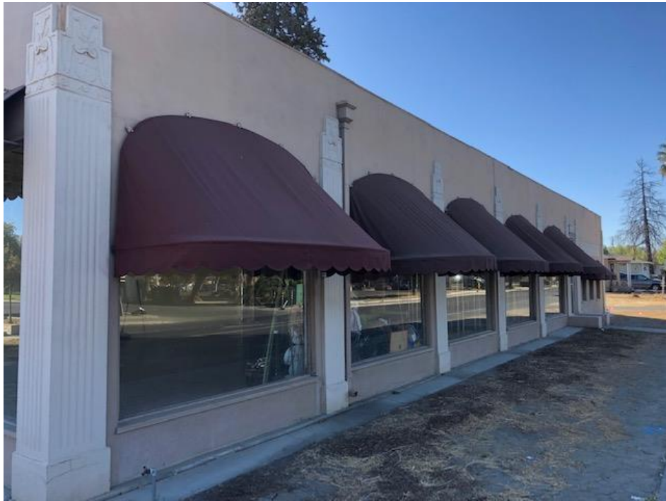
Photograph 3 View looking south from West Street at the west elevation of 2 Main Street. Note that the cloth awnings cover the groups of transom windows.
