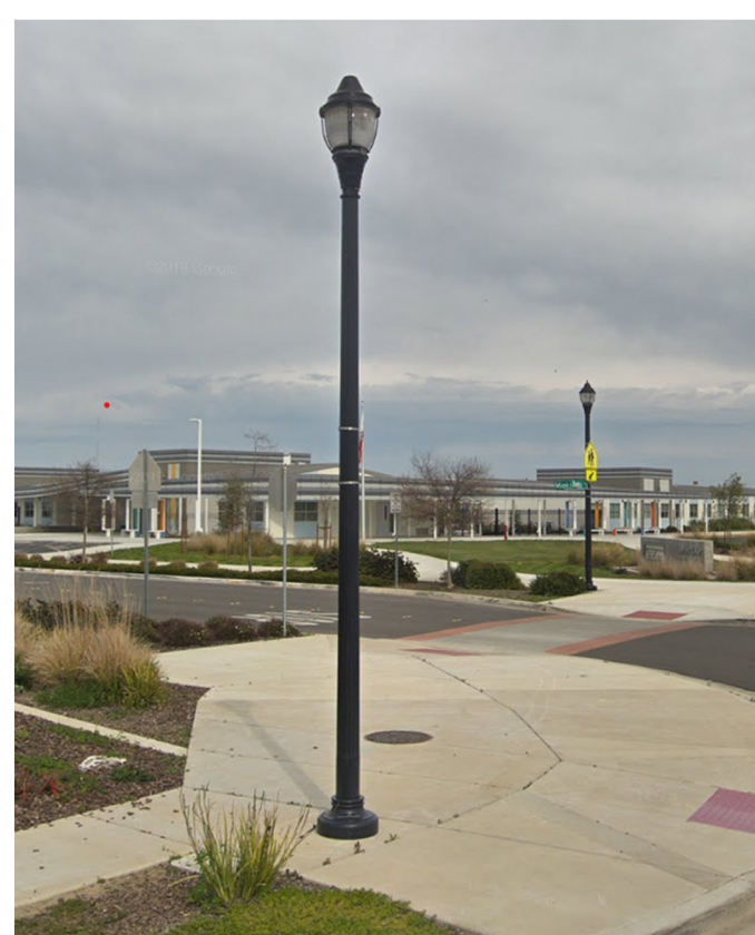
TYPICAL STREET LIGHT
