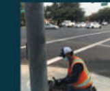
Court Street Improvements
