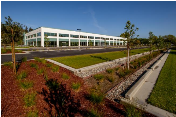
Low impact development techniques including bioswales allow for the collection and filtration of stormwater runoff.
