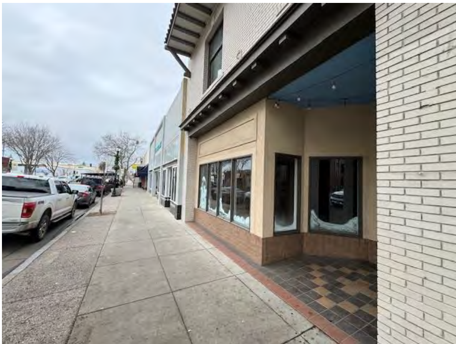
Photograph 8: Similar view as Photograph 7, but looking west down Main Street.
