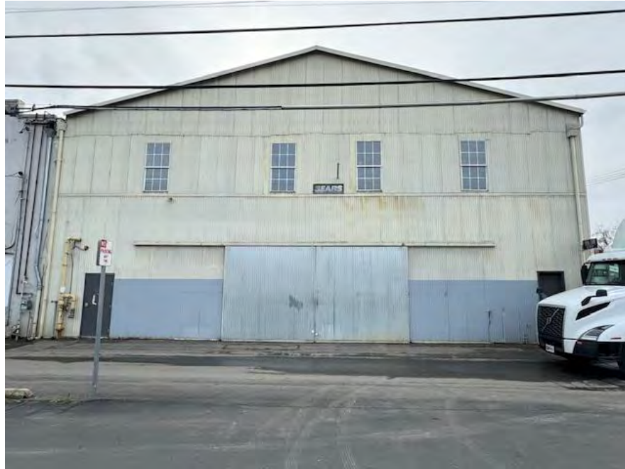
Photograph 9: View looking south from Dead Cat Alley towards the front of the former Fashion Stable building and now the rear of the Roth Building that shares a common wall with 350 College Street.
