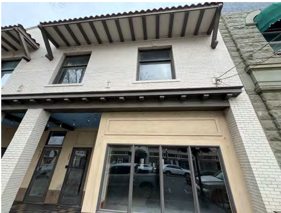
Photograph 6: View looking north at the altered windows on the first floor and what was likely once a clerestory window above the lower picture windows.
