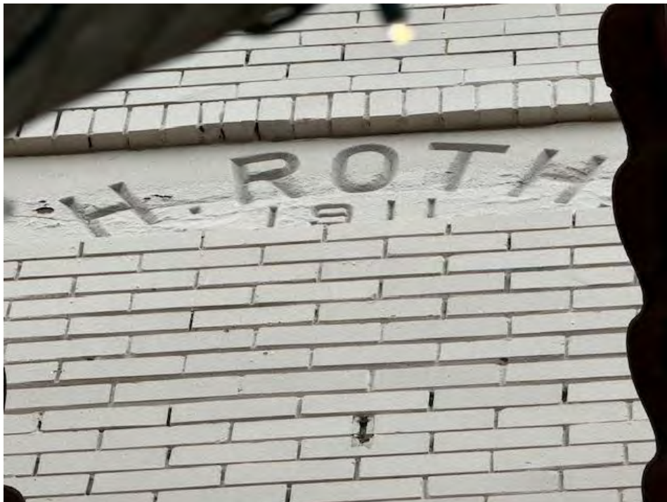
Photograph 4: View looking at the marquee set in the brick below the parapet that reads "H. ROTH 1911."
