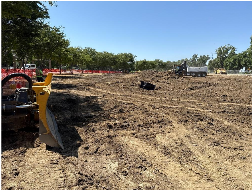
Grading of the site for the Parking Lot project
