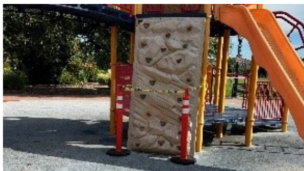
New rock climbing wall installed at Jack Slaven Park.
