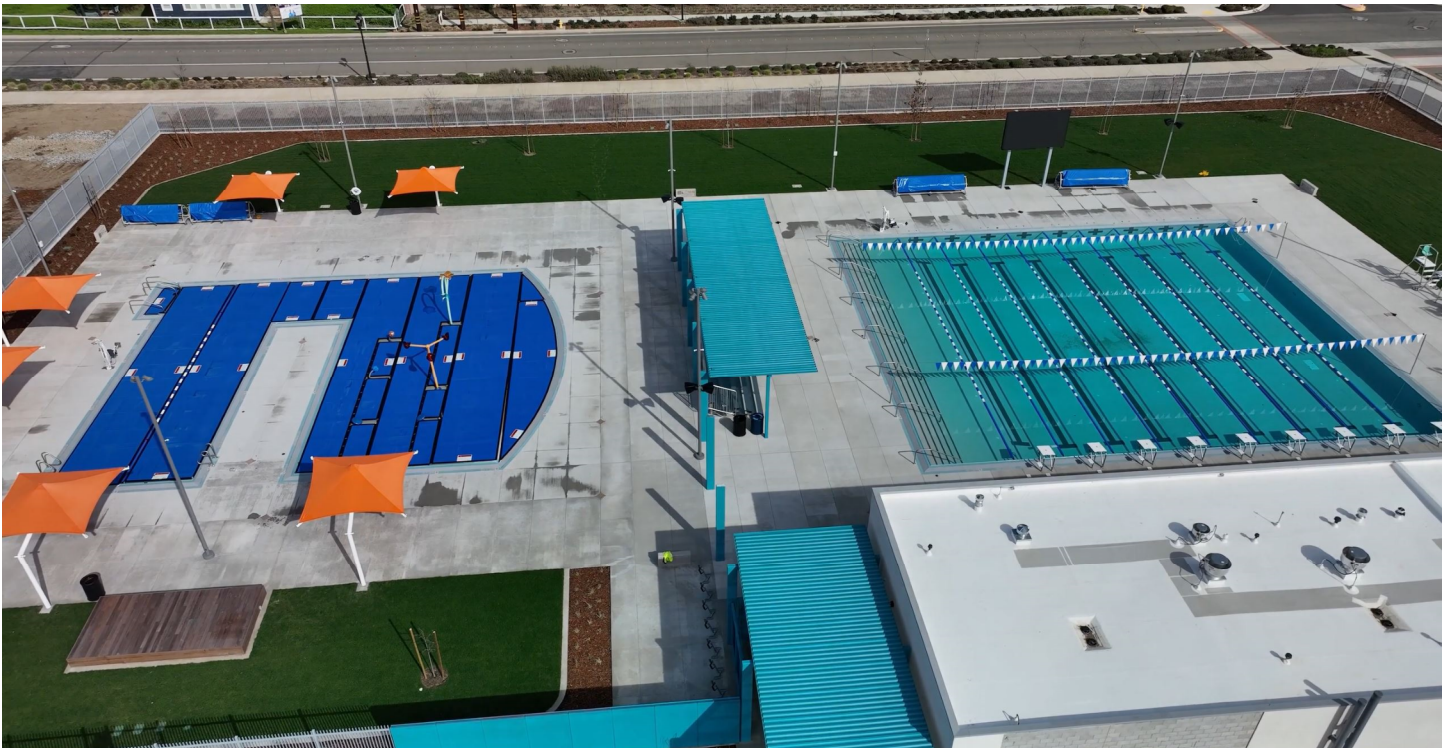
Drone Photography (February 2026)
