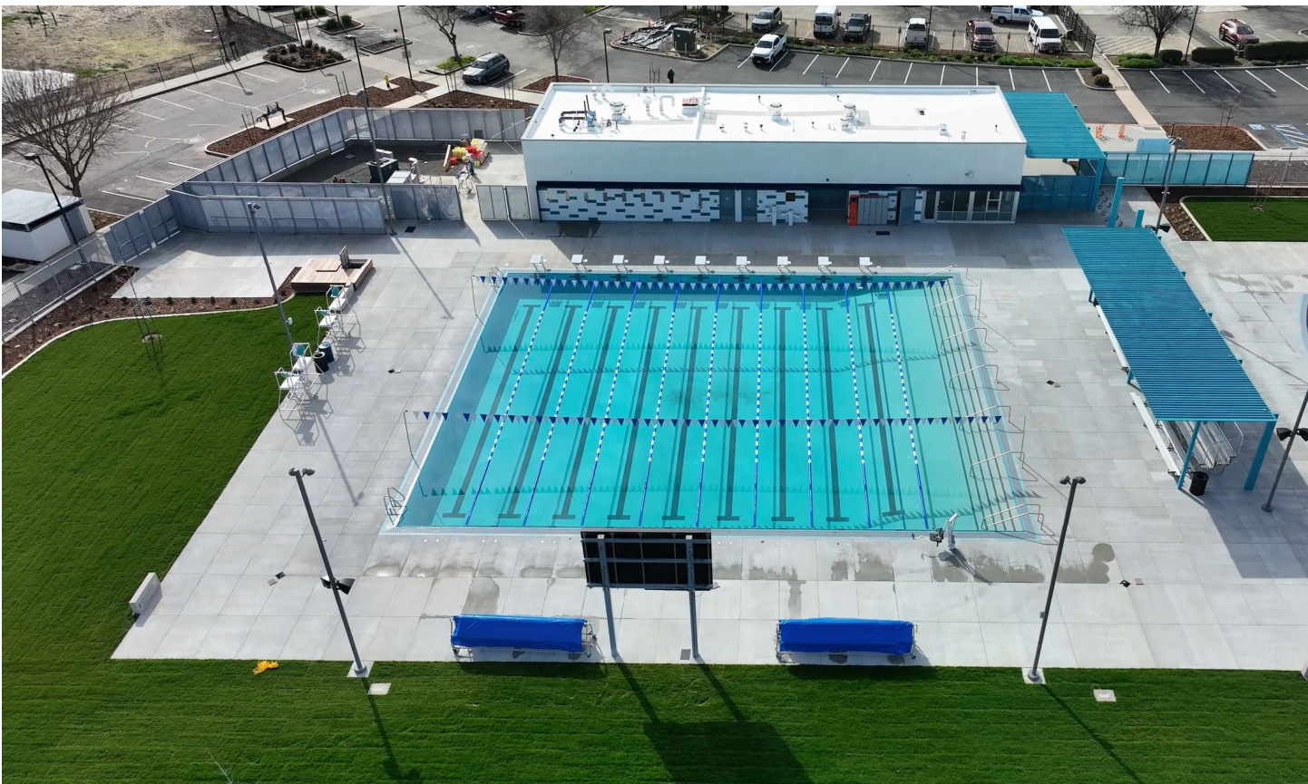
Drone Photography (February 2026)
