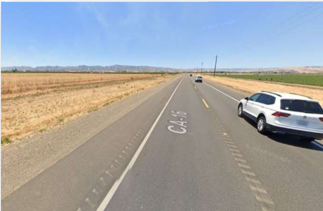
Figure 2: CA-16 Westbound Existing Condition
