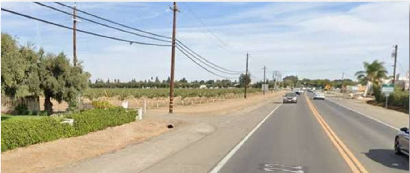
Figure 21: SR-16 Eastbound Approaching County Road 98 Existing Conditions
