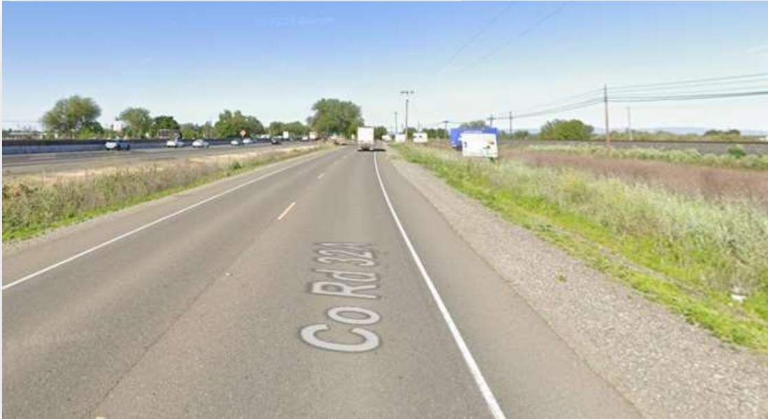
Figure 15: County Road 32A Existing Conditions
