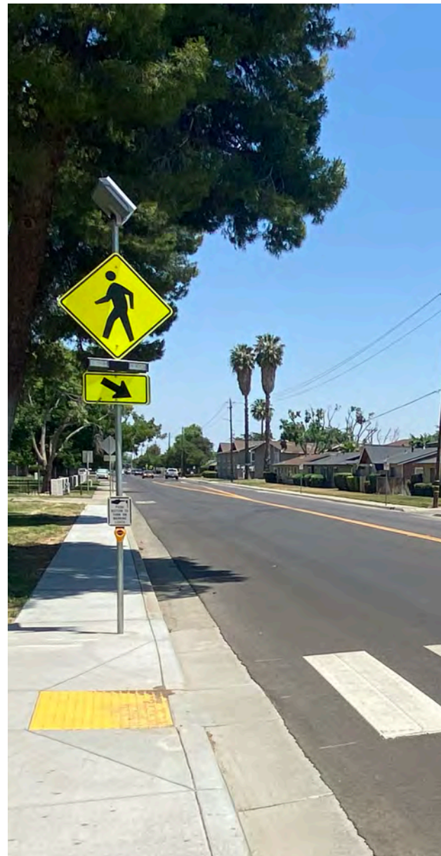
Figure 40: Rectangular Rapid Flashing Beacon
