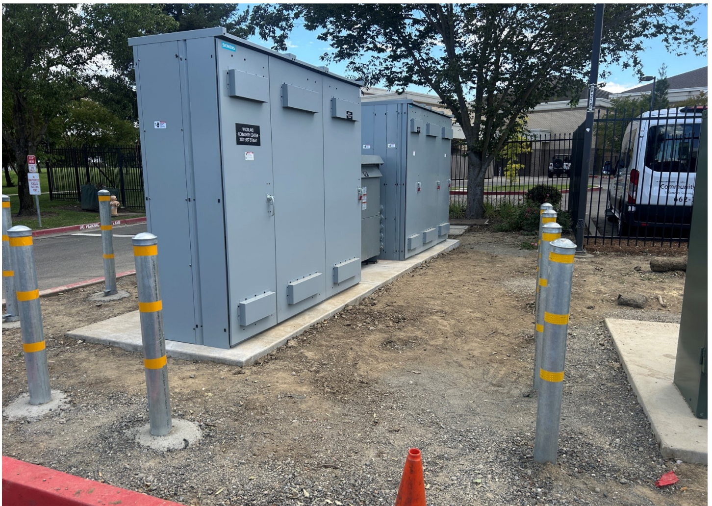
Switchgear Installation (May 2026)
