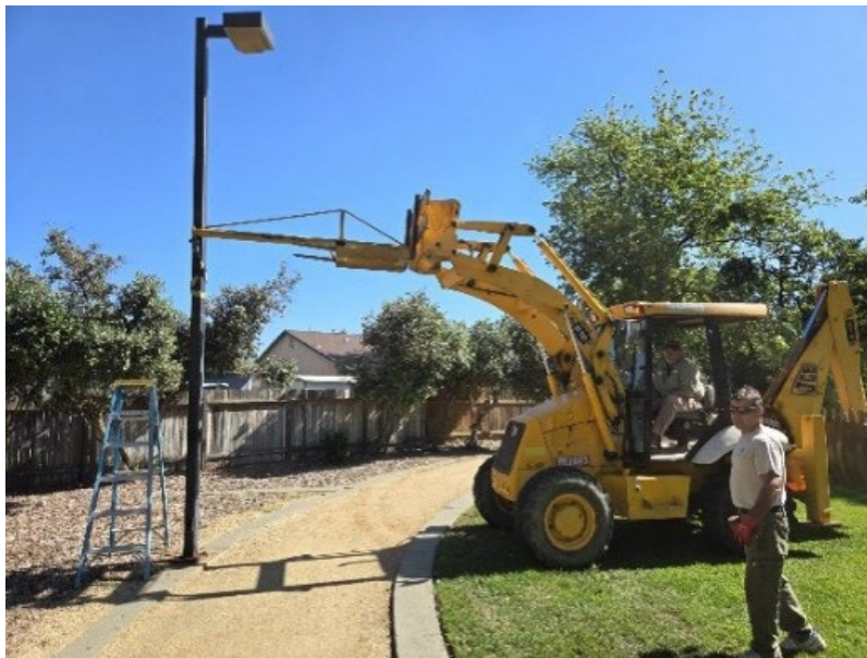
Light pole replacement at Schneider Park
