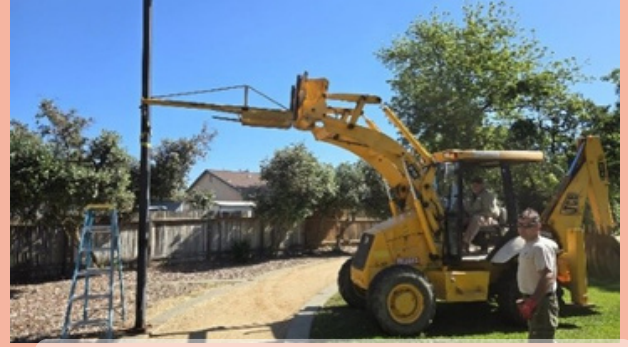
Replaced several light poles at Cline Park
