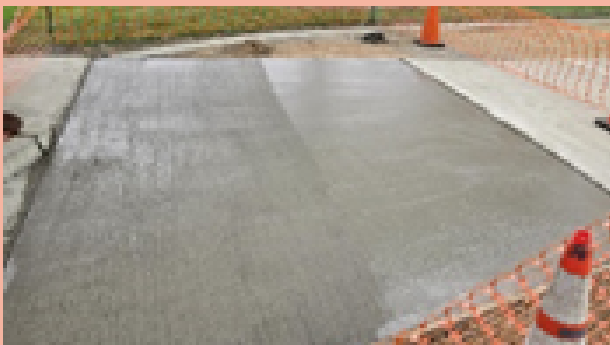
Repaired entrance at Cline park
