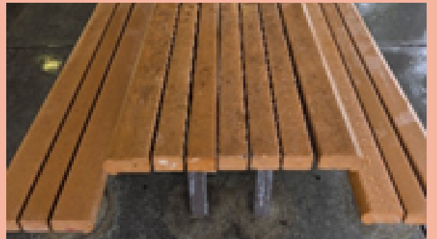
Repaired Pioneer Park tables
