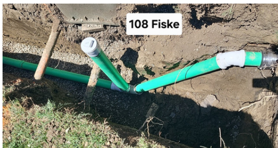
2026 Water & Sewer Replacement Project Construction
