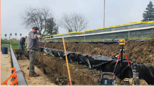
Repaired first level of Brooks' retaining wall
