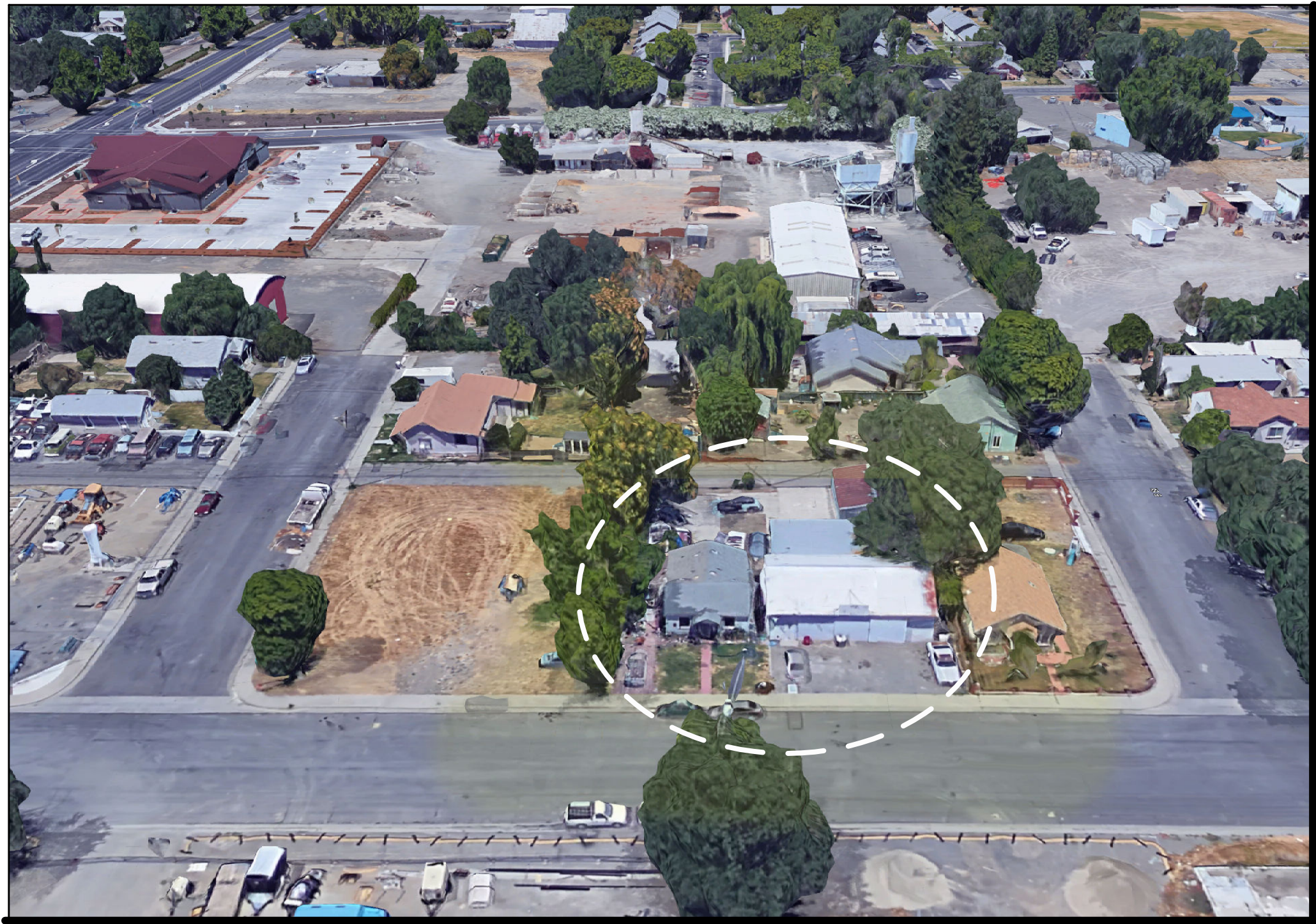
EXISTING SITE CONTEXTUAL PHOTO
